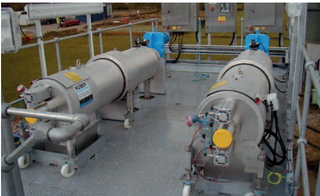
STRAINPRESS® with heatable casing pipe
