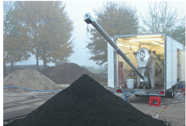
Contract dewatering with a trailer-mounted HUBER Screw Press Q-PRESS®
