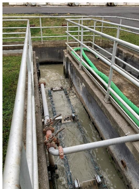
Grit Channel with Chain and Bucket
