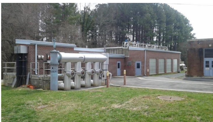
DN Filter Pump Station (left) and DN Filter Facility
