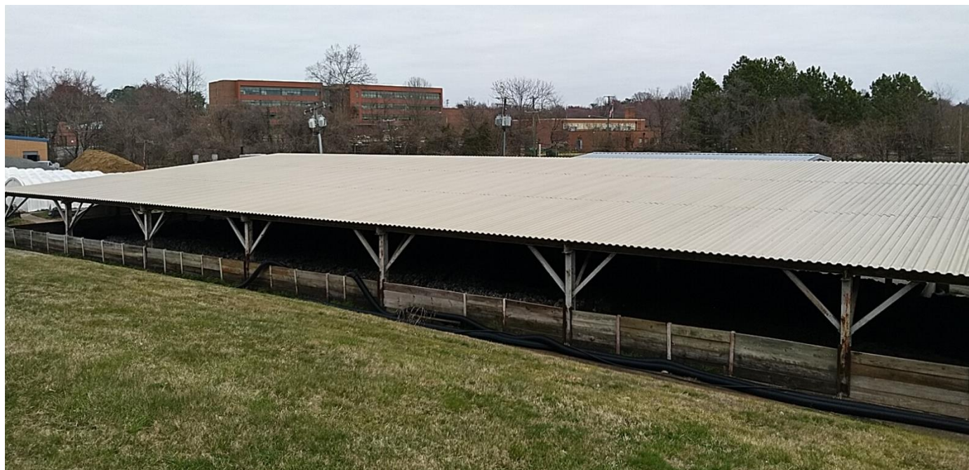
Biosolids Storage (back-end view)
