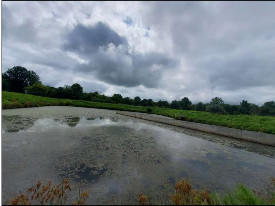
17 - View of stormwater pond located to the southwest of the site
