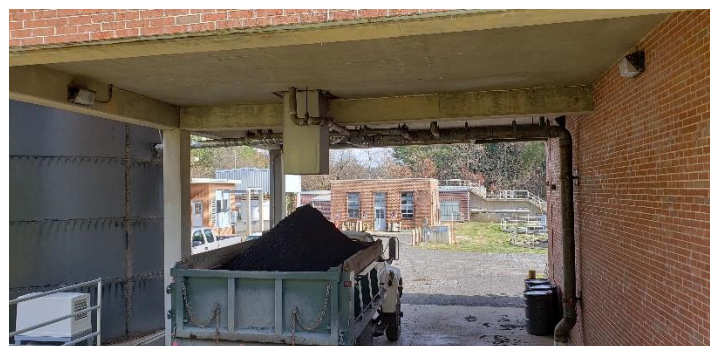
Dewatered Cake Transfer to On-Site Storage
