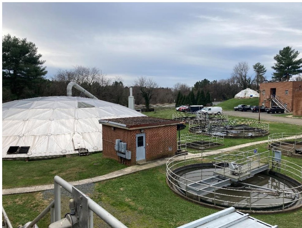
Primary Clarifiers (with sludge pumping station) and former Trickling Filter (covered)
