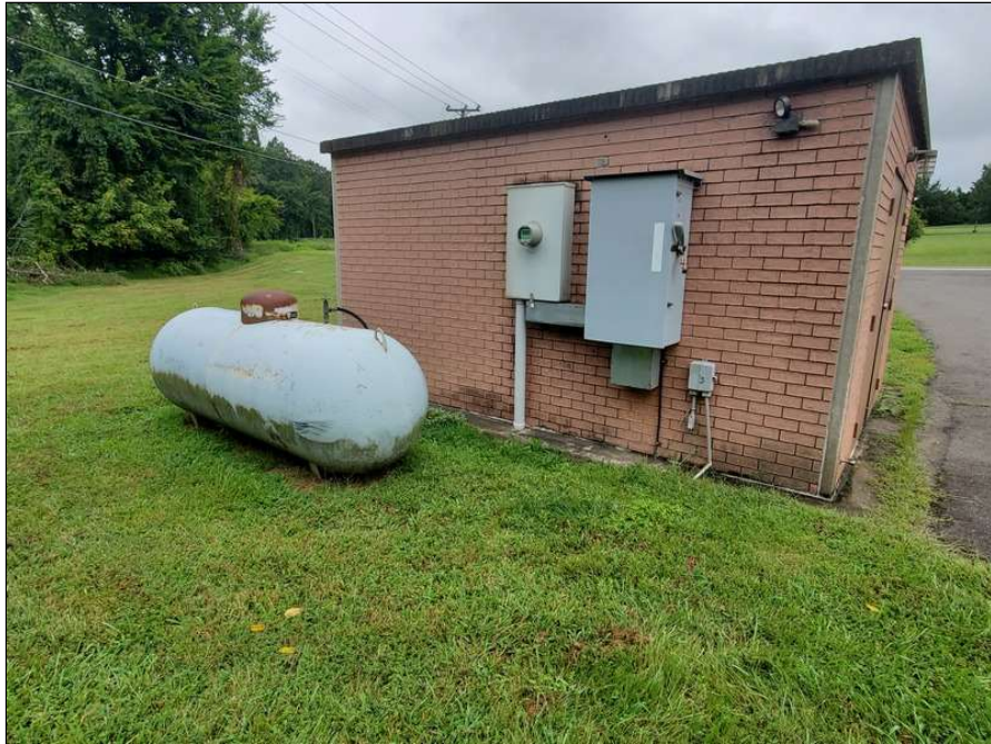
8 - Rear of utility shed
