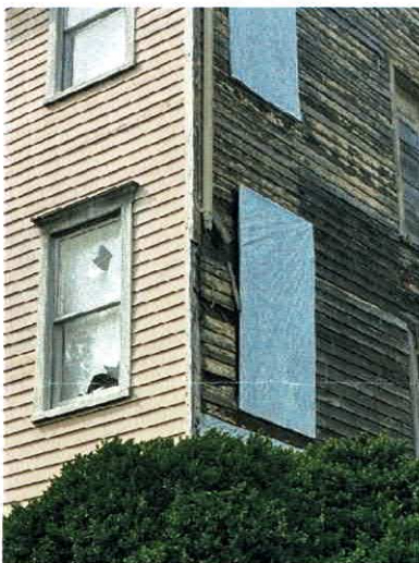
(Picture 9: Shows inadequate roof Drainage, rotted wood And broken windows)
