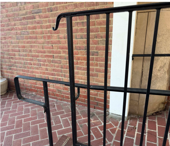
02 PRECEDENT - IRON RAILING
