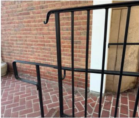
02 PRECEDENT - IRON RAILING
