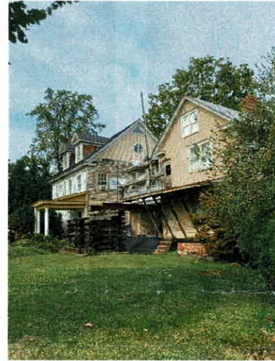
(Picture 3: Shows faulty structural supports, Inadequate roofing on right side, wood rot, and peeling paint)
