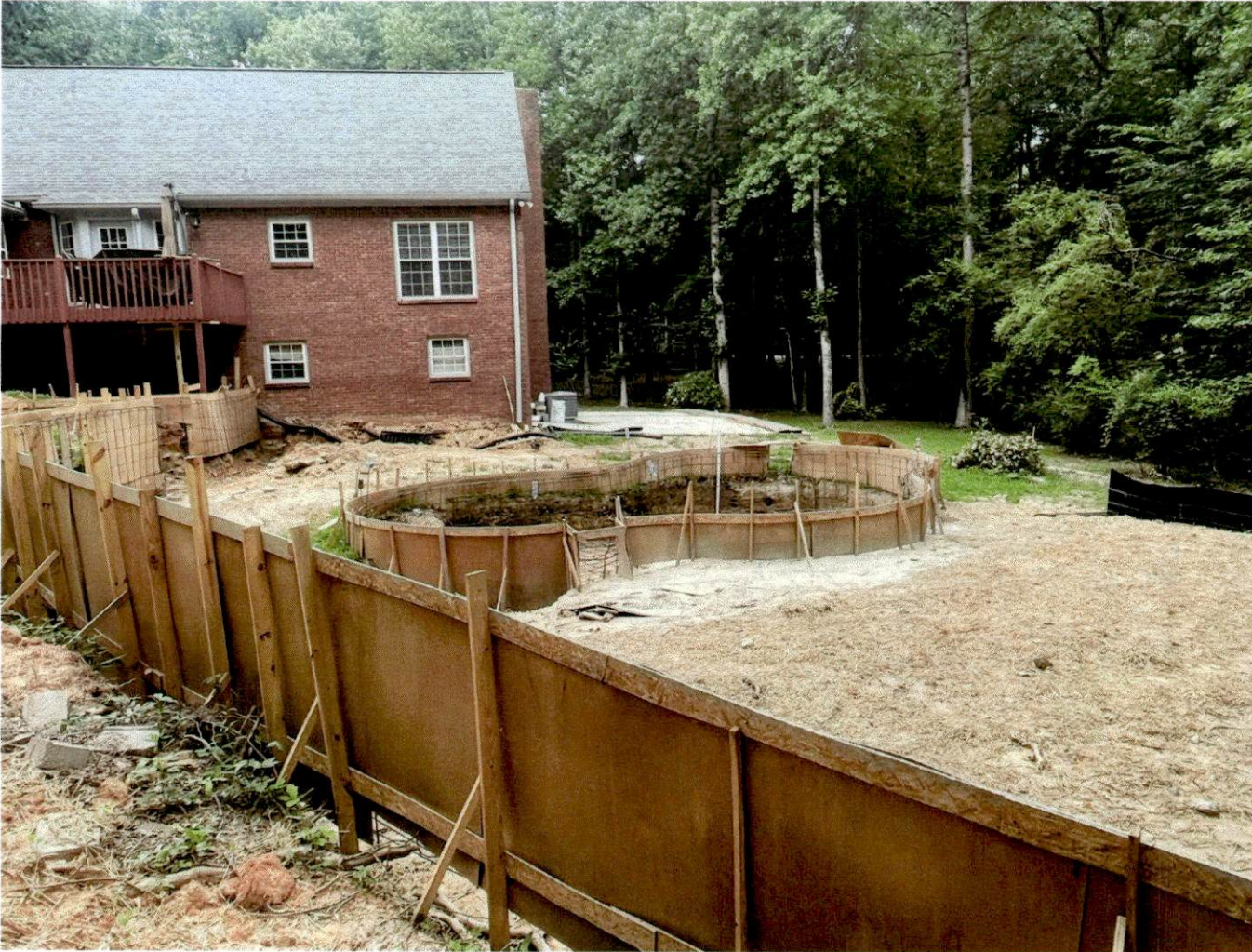
View of retaining wall and back side of the pool.
