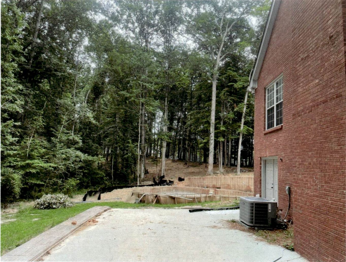
View showing existing driveway and how it ties into the pool location.
