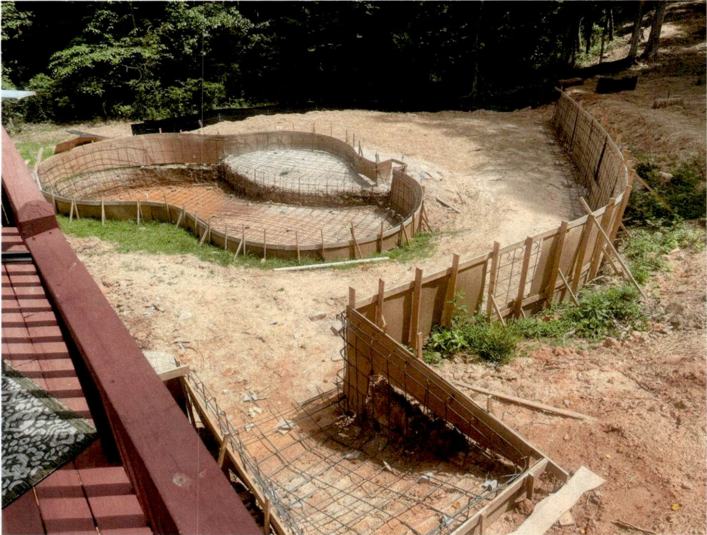
View from upper deck showing grading, framing and rebar installation.
