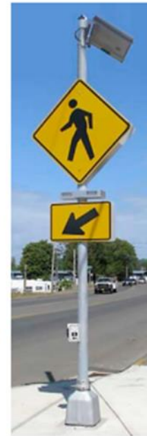
Wrap-around RRFB Light Bar with Required Signage
