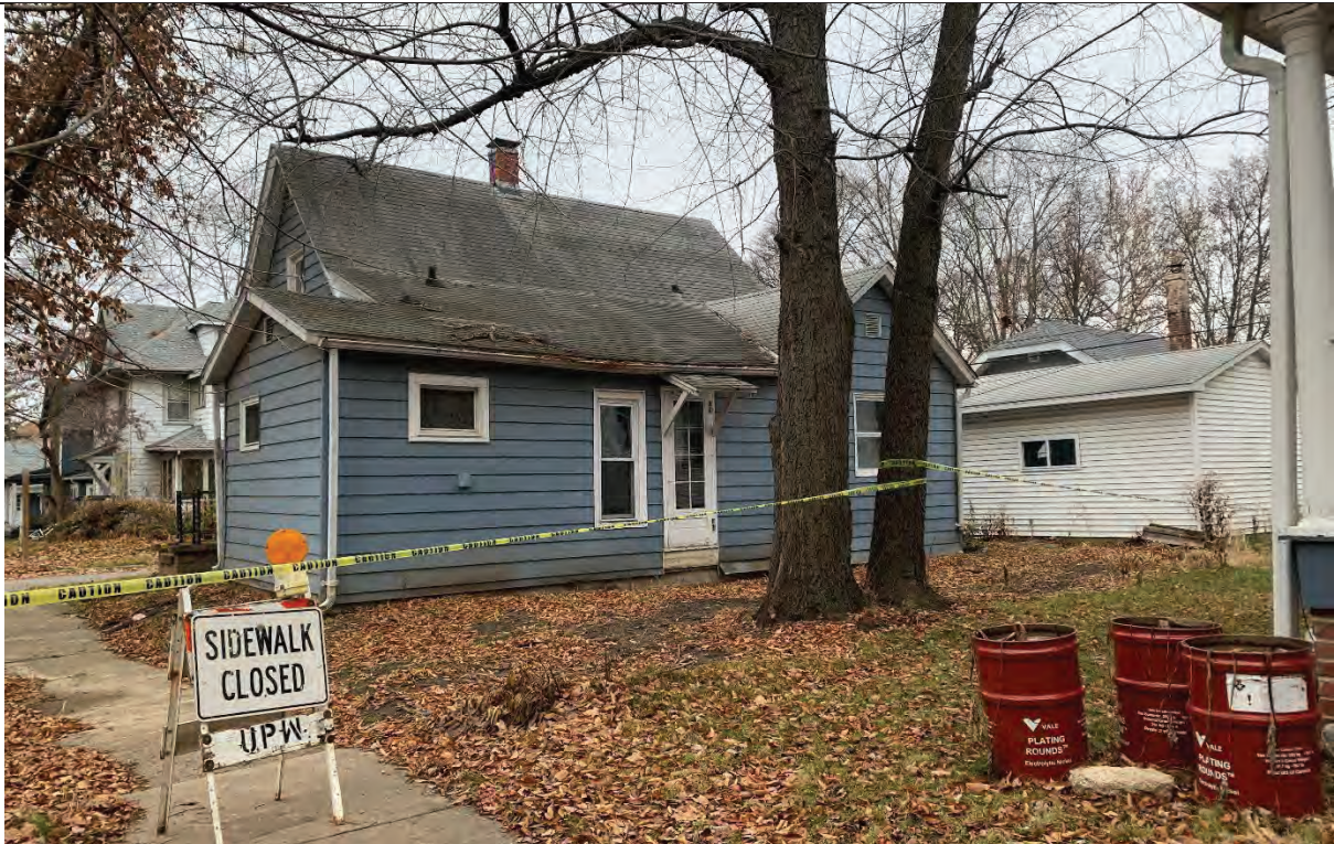
Figure 4. Illinois Street, facing northwest (note "building condemned" caution tape).
