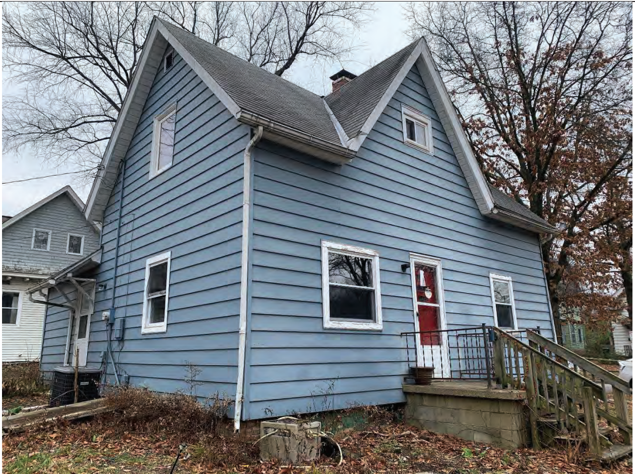
Figure 3. Illinois & Birch Streets, facing northeast (closeup).
