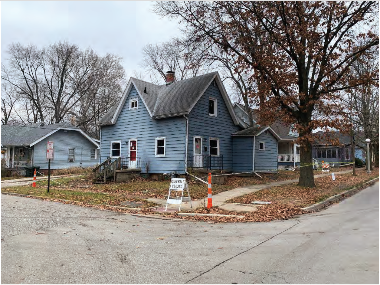
Figure 1. W. Illinois & Birch Streets, facing northeast.
