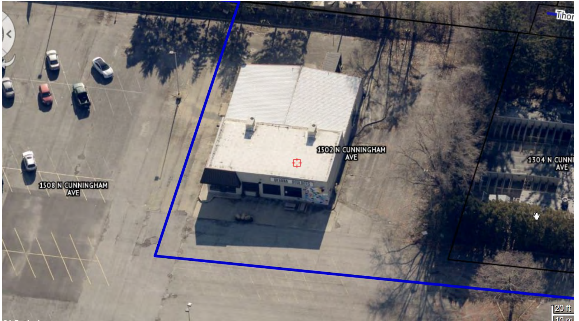
FIG. 2: 2021 AERIAL – LOOKING SOUTHc
