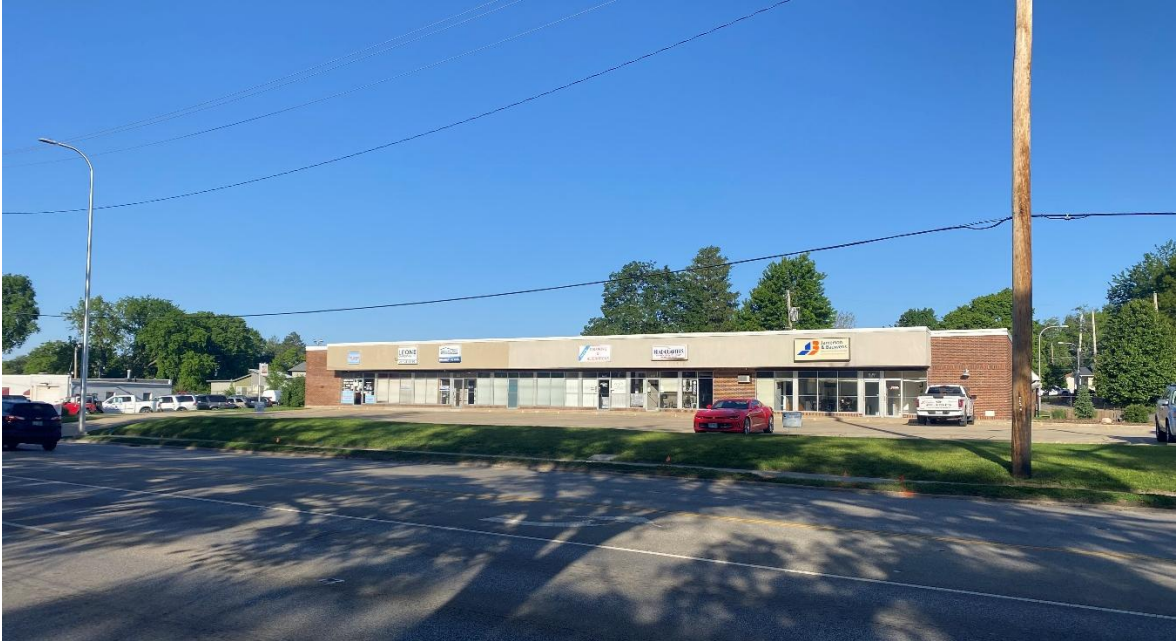
View towards 909 N Cunningham Avenue (“Apple Tree Plaza”) directly across North Cunningham Avenue.
