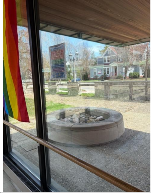
French drain at the Urbana Presbyterian Church, A. Richard Williams Architect, April 2026 by Phyllis Williams
