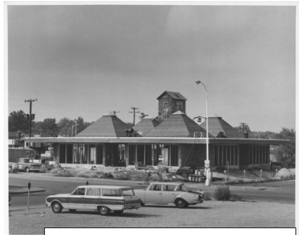
Under construction with the feed store behind. From the Champaign County Archives, vertical file
