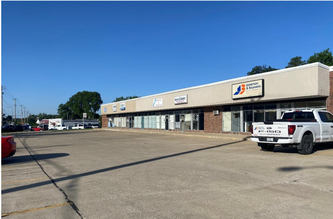
View of 909 N Cunningham Avenue (“Apple Tree Plaza”) from the parking lot.
