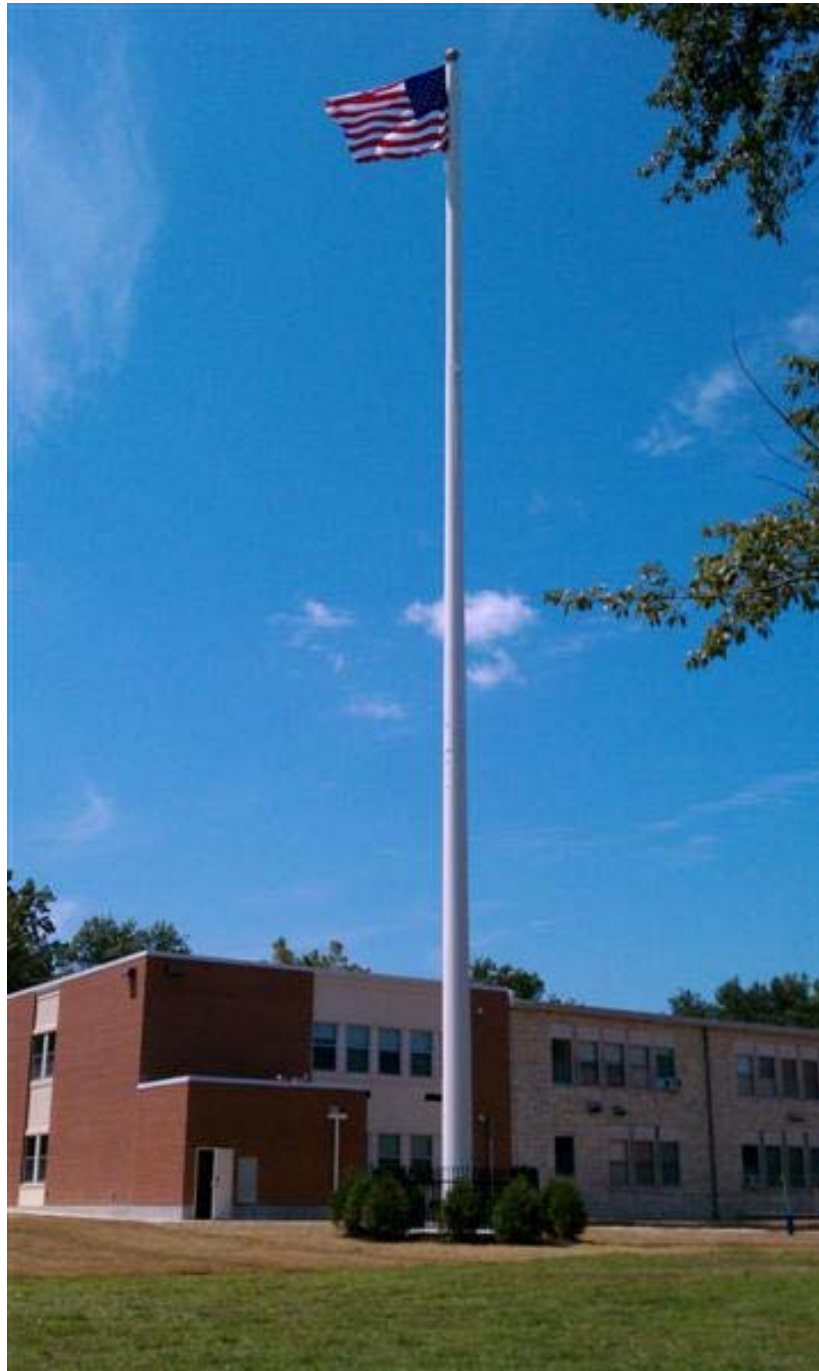
Similar monopole telecommunications tower now sited on a school property in Quincy, Illinois
