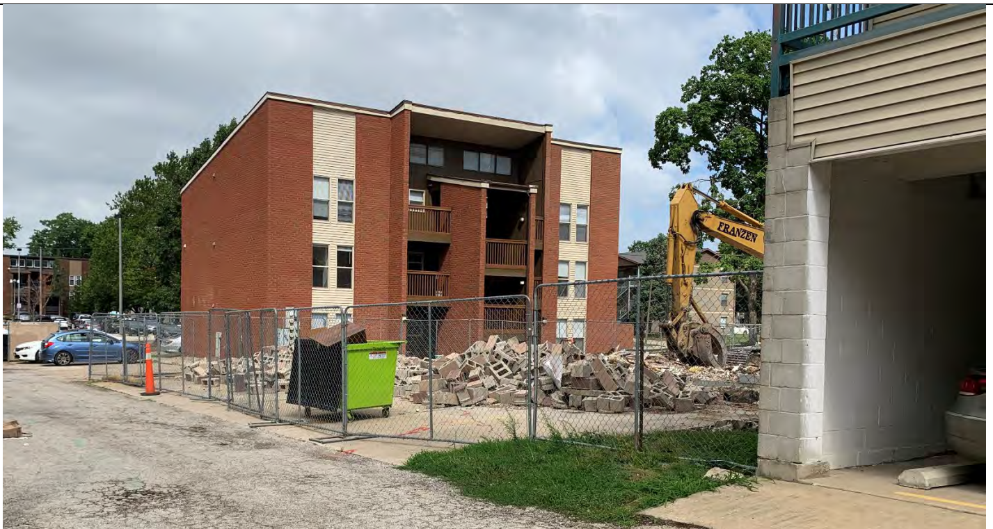
Fig. 2: Looking northwest: note extent of parking spaces
