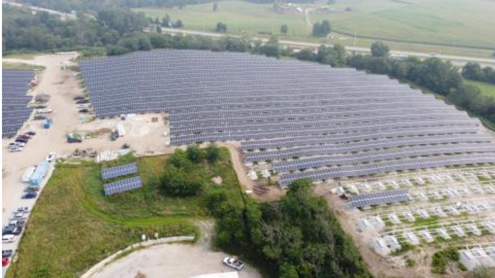
City of Urbana Community Solar Array
