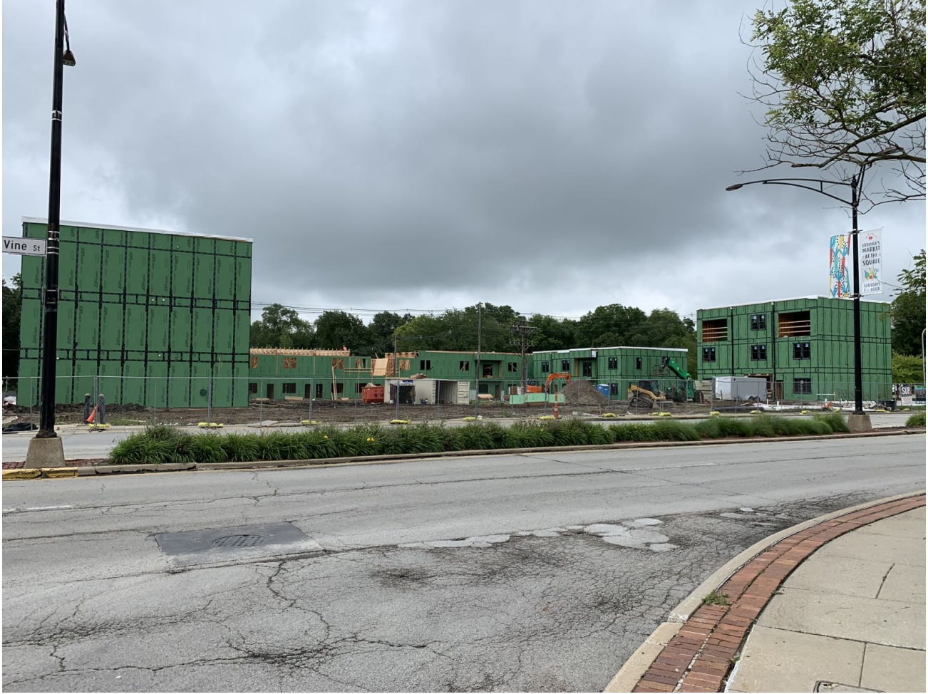
200 South Vine Street townhomes under construction (2020)
