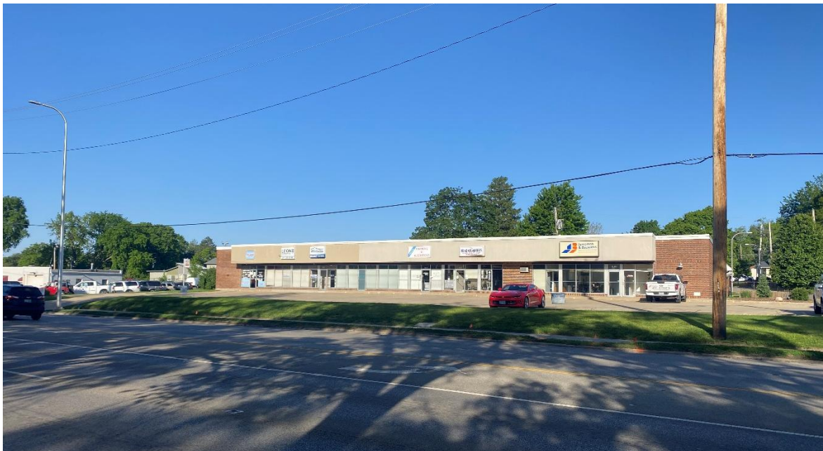
View towards 909 N Cunningham Avenue ("Apple Tree Plaza") directly across North Cunningham Avenue.
