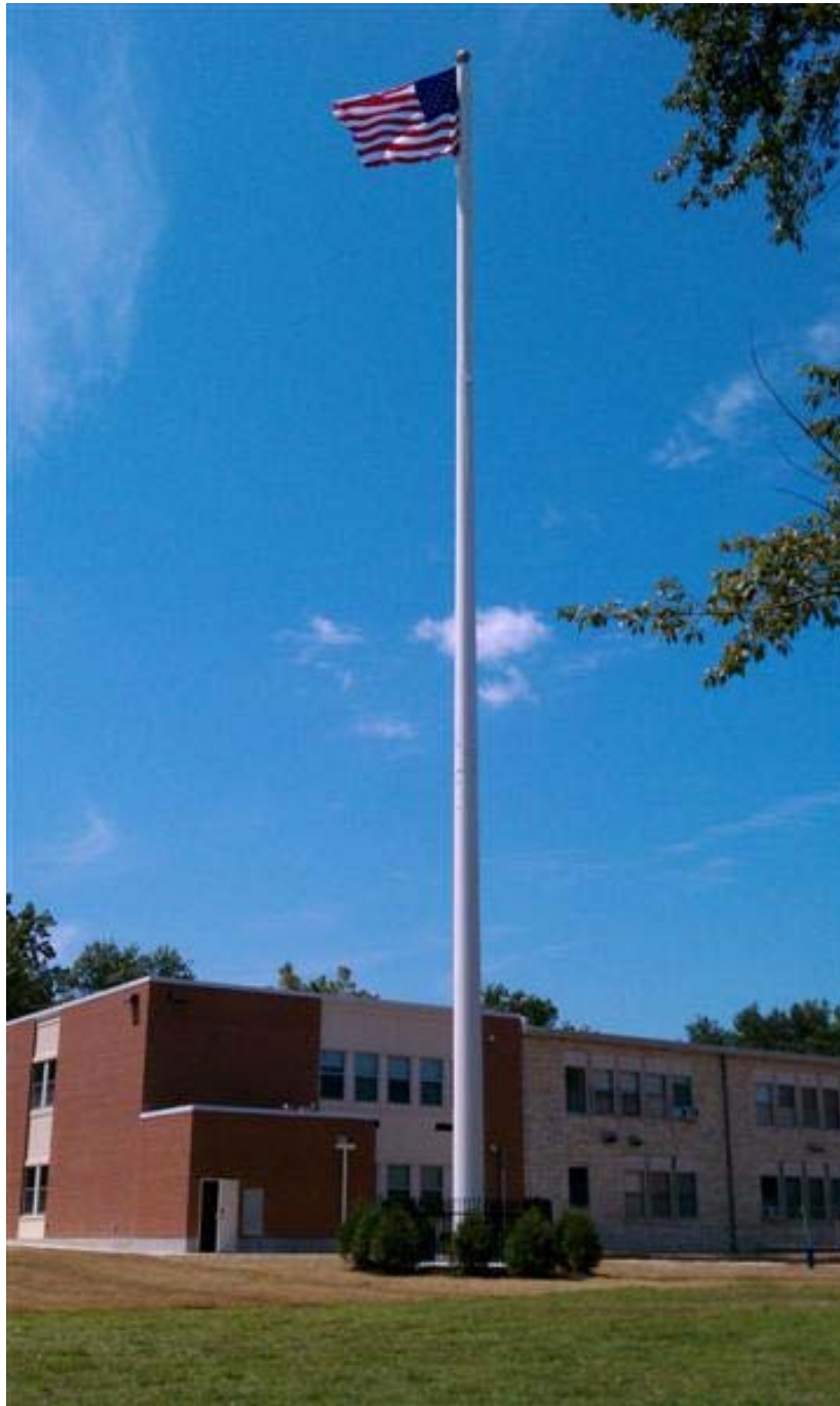
Similar monopole telecommunications tower now sited on a school property in Quincy, Illinois
