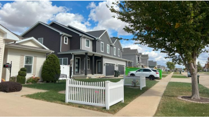
Current: E Lexington Dr, Urbana, IL (Duplexes and SF Detached Homes - Suburban pattern)
