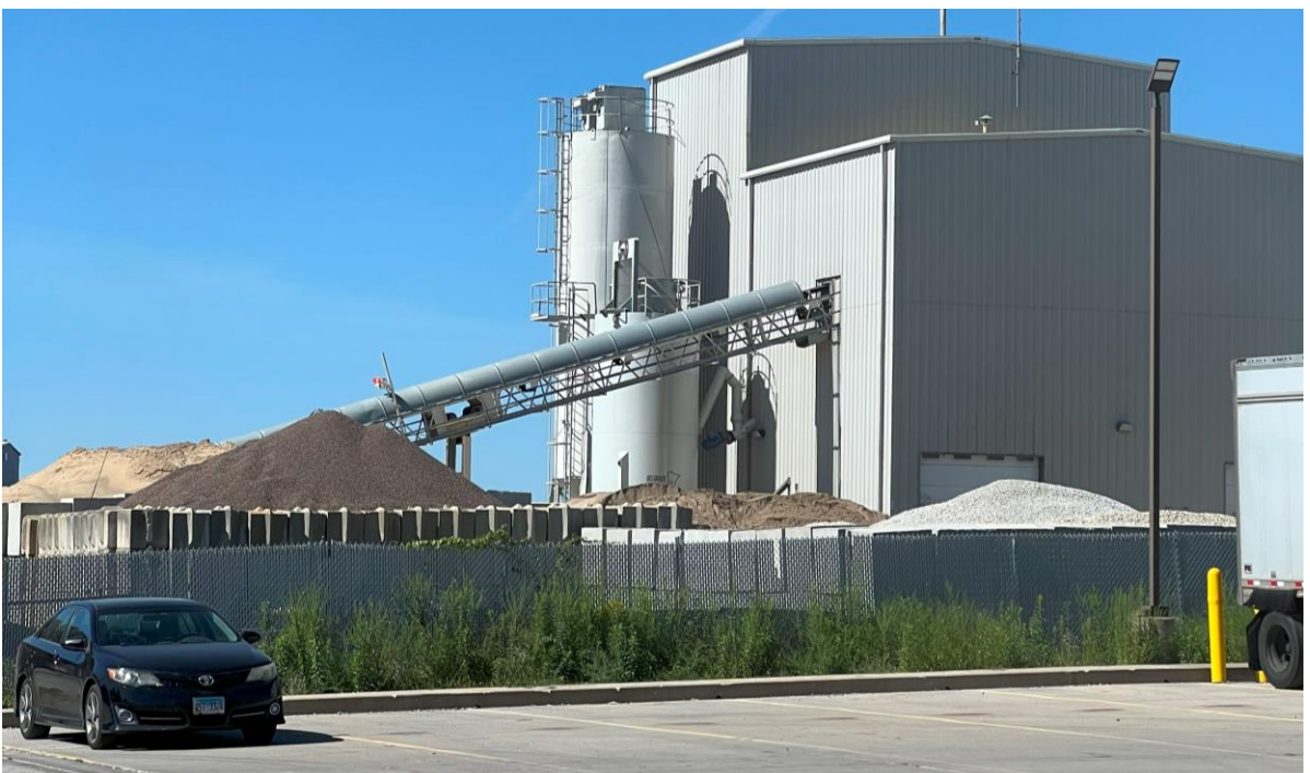
Current: 2766 N Lincoln Ave in North Urbana
