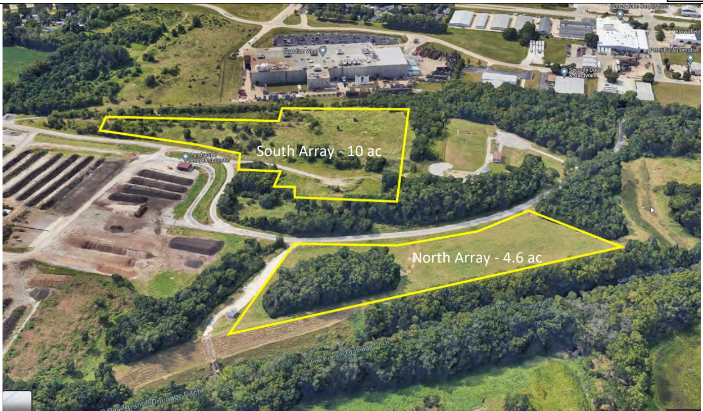
Figure 1. Project site from north (GoogleMaps)
