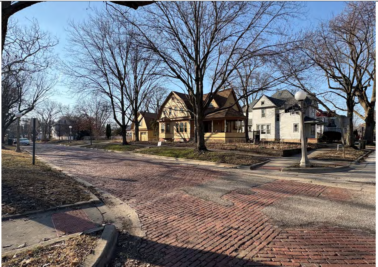
Figure 4. From southeast – intersection
