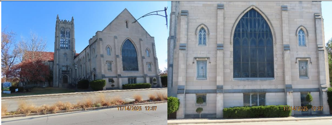
Detail of Western-Facing Façade
