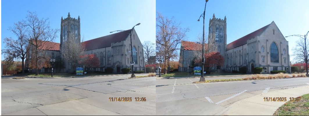
The intersection of Race Street and Green Street, Looking South
