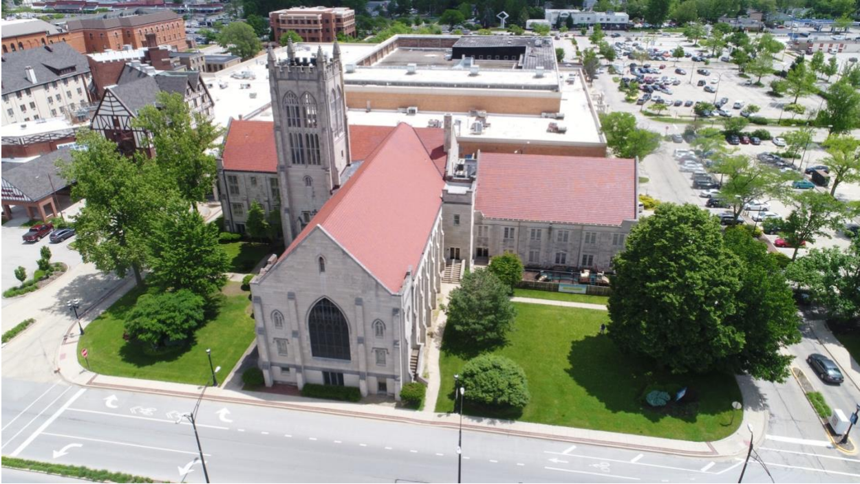
Aerial images of the current building, courtesy of Renaissance Roofing
