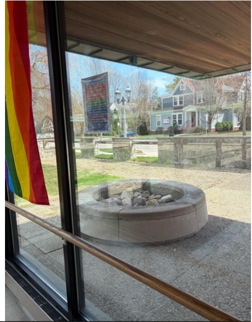
French drain at the Urbana Presbyterian Church, A. Richard Williams Architect, April 2026 by Phyllis Williams
