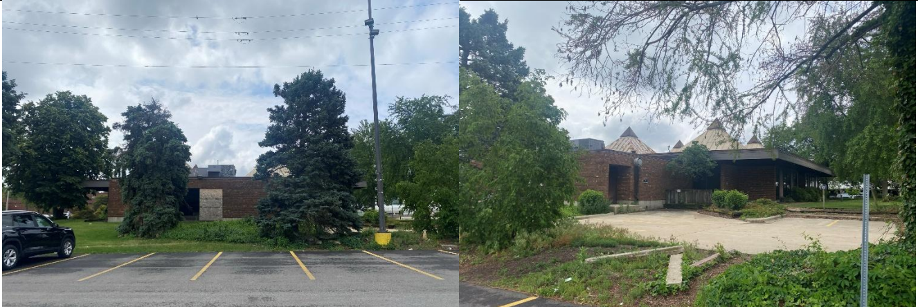
View of the north façade and the northwestern corner.
