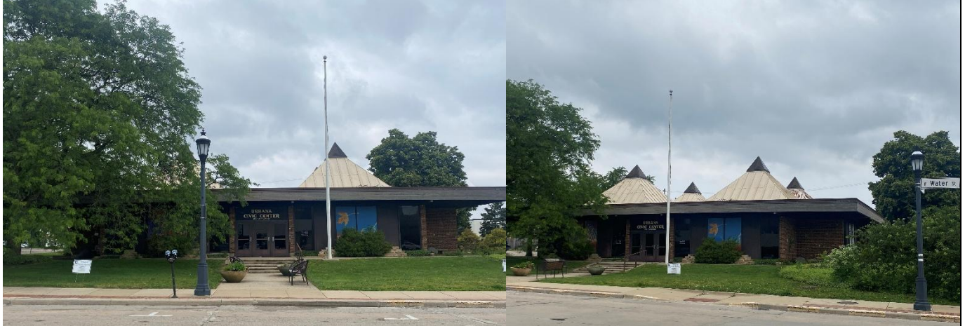
View from Water Street of the south façade.
