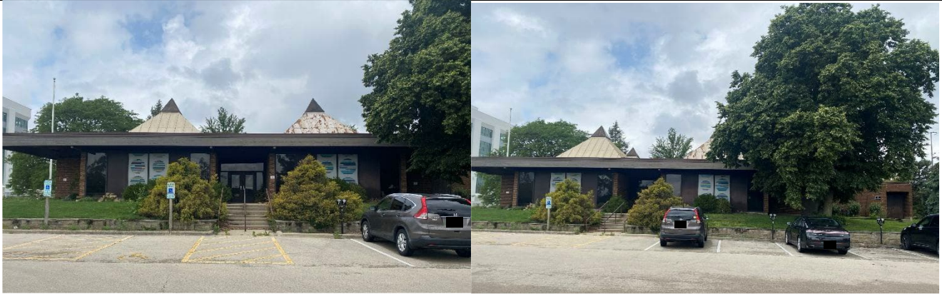
View of the east façade, featuring the main block of the building (left) and the back wing (right).
