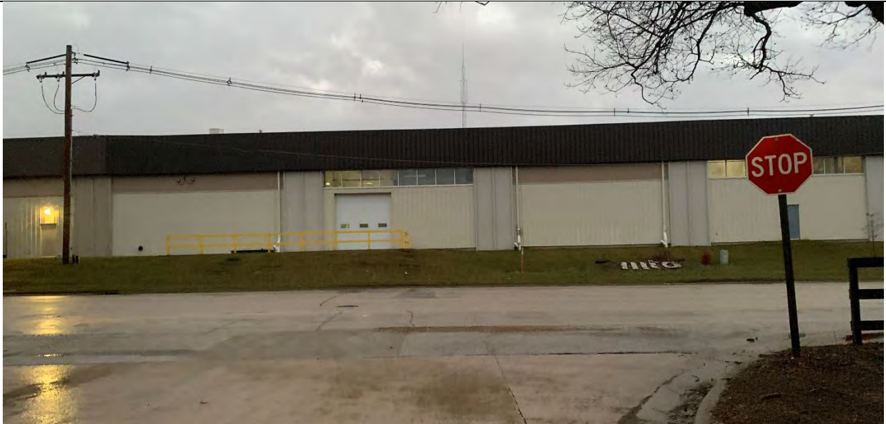
Fig. 4: Looking south at Ash Street intersection at CUMTD building
