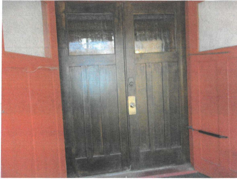
Façade/North elevation, west side. Entrance doors.
