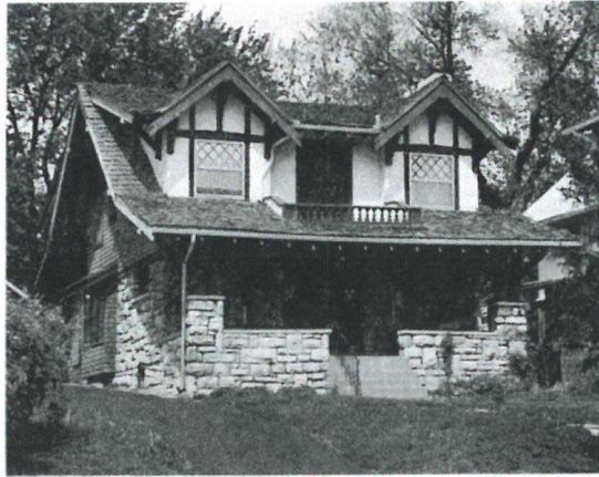
Craftsman designed house with stucco, half-timbering and stone elements (McAlester and McAlester 2005:461)
