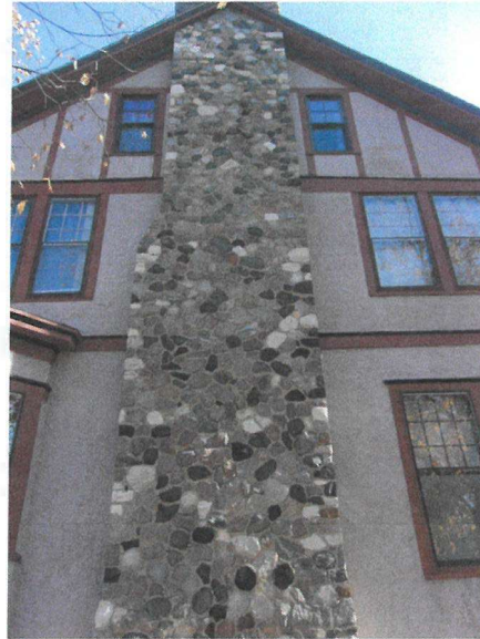
West elevation. Chimney details.
