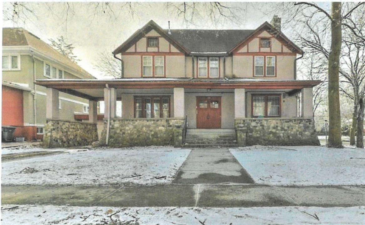
Photograph of the Huff House in 2022. View to the southwest (top) and south (bottom).
