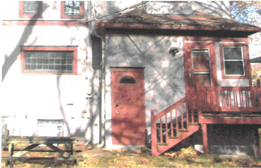
South elevation, first floor, center and east end. Center: smooth stucco water table, glass block basement window, and 23 light fixed sash window. East end: basement door and stairway to back porch and access to pantry/kitchen.
