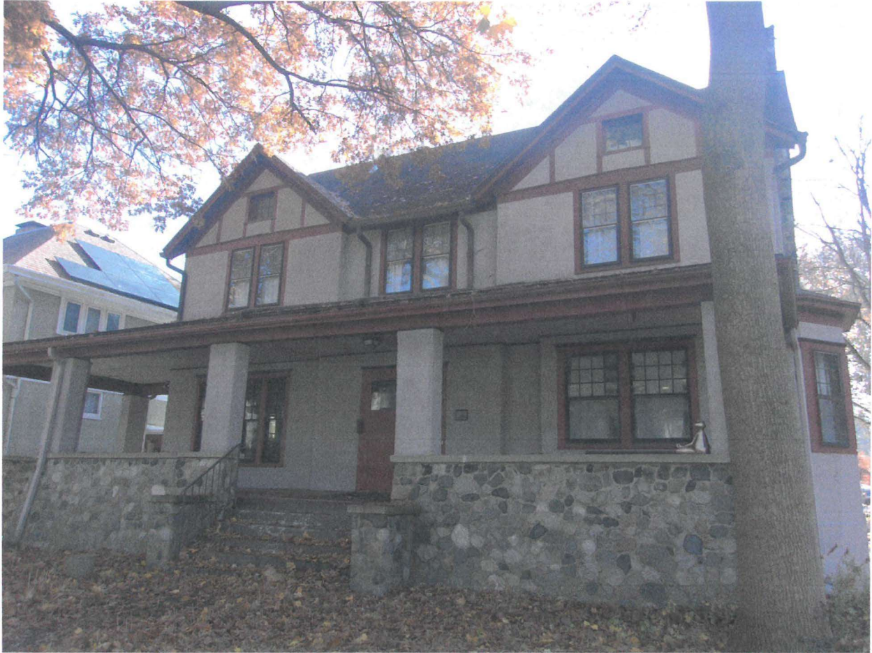
Façade/North elevation. View to southeast.
