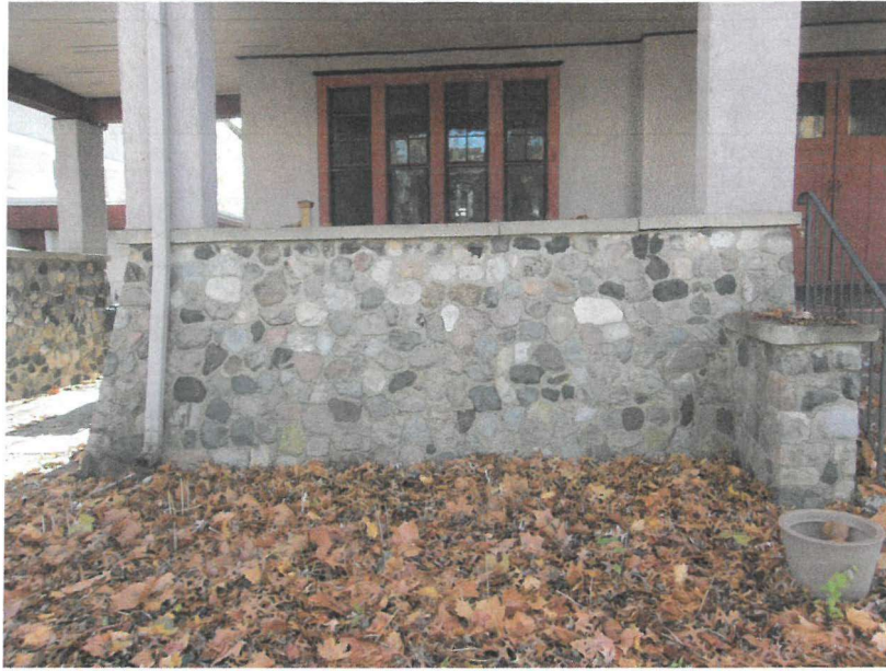
Façade/North elevation. Porch details.
