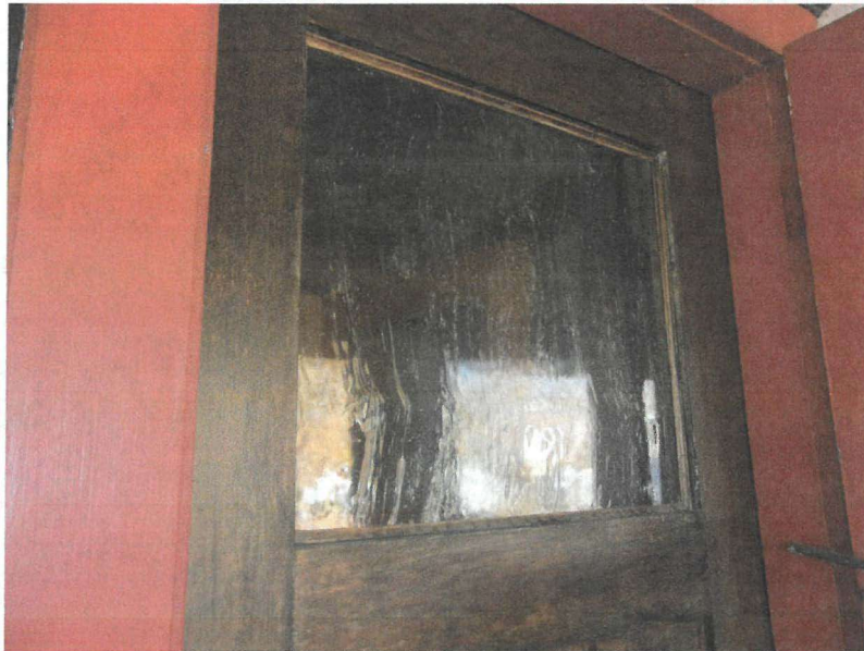
Façade/North elevation. Entrance door detail. Glazed panel of “cylinder glass”.
