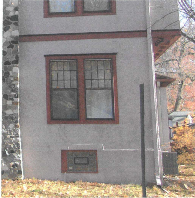
West elevation, first story, south end. 12/1 light sash windows, smooth stucco water table and glass block basement window.
