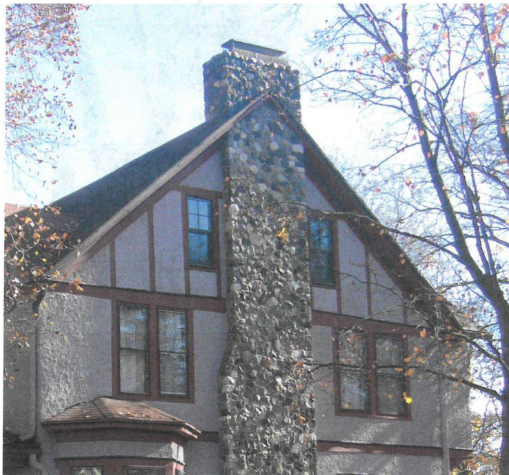
West elevation, detail, second and top story.
