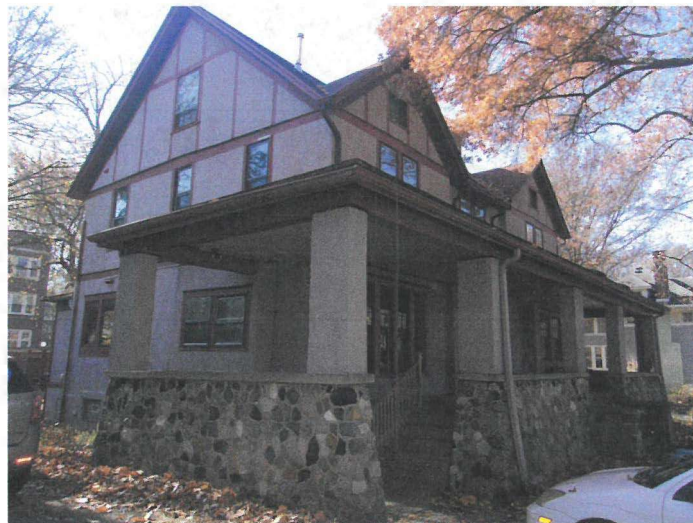
East and north elevations: porte-cochere.
