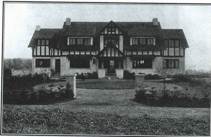
THE CRAFTSMAN HOUSE ESPECIALLY DESIGNED FOR MR. F. S. PEER OF ITHACA, N. Y. AN INTERESTING EXAMPLE OF STUCCO AND HALF-TIMBERING CONSTRUCTION.
