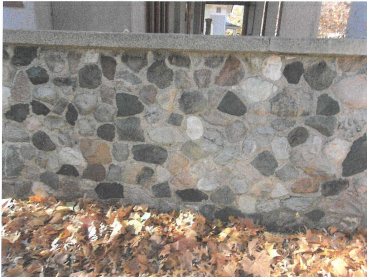
East elevations: porte-cochere, detail of split/unsplit cobblestones.
