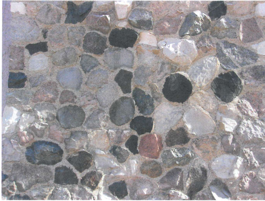
West elevation. Chimney details, split and unsplit cobblestones.
