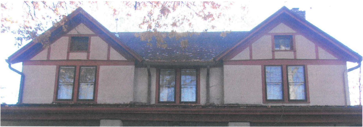
Façade/north elevation. Second and upper story details.
