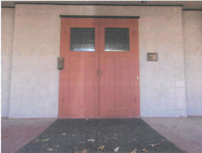
Façade/North elevation, west side. Entrance, storm doors.
