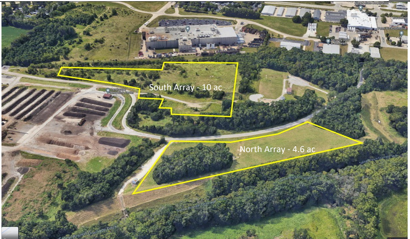
Figure 1. Project site from north (GoogleMaps)
