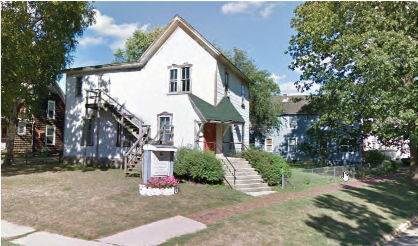
Fig. 4: Photo of former church (Google Streetview, 2017).
