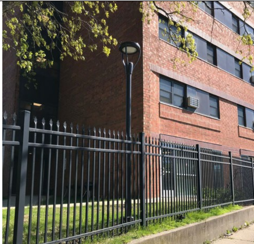
Fig. 10: Fence and lighting along Harding Drive
