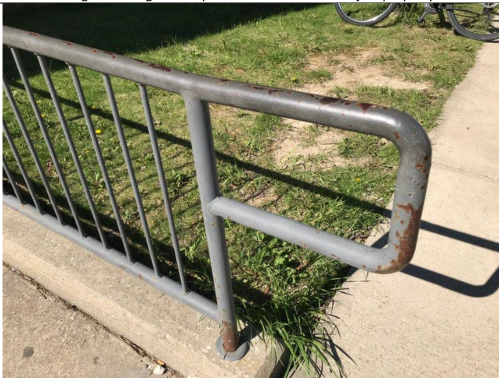
Fig. 6: Handrail at North property entrance
