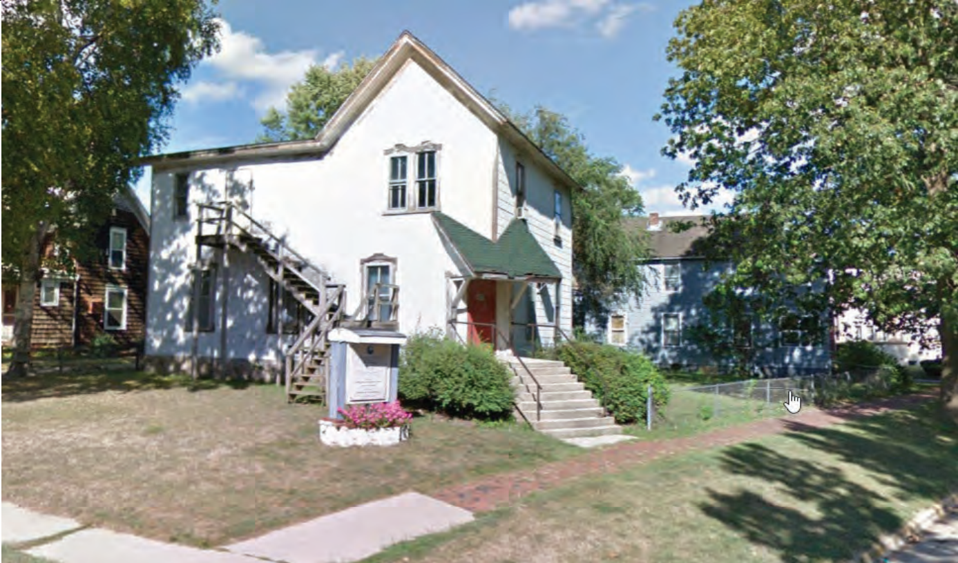
Fig. 4: Photo of former church (Google Streetview, 2017).
