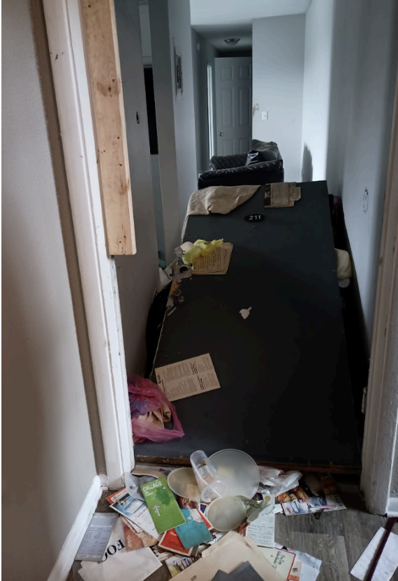
Broken down doors
