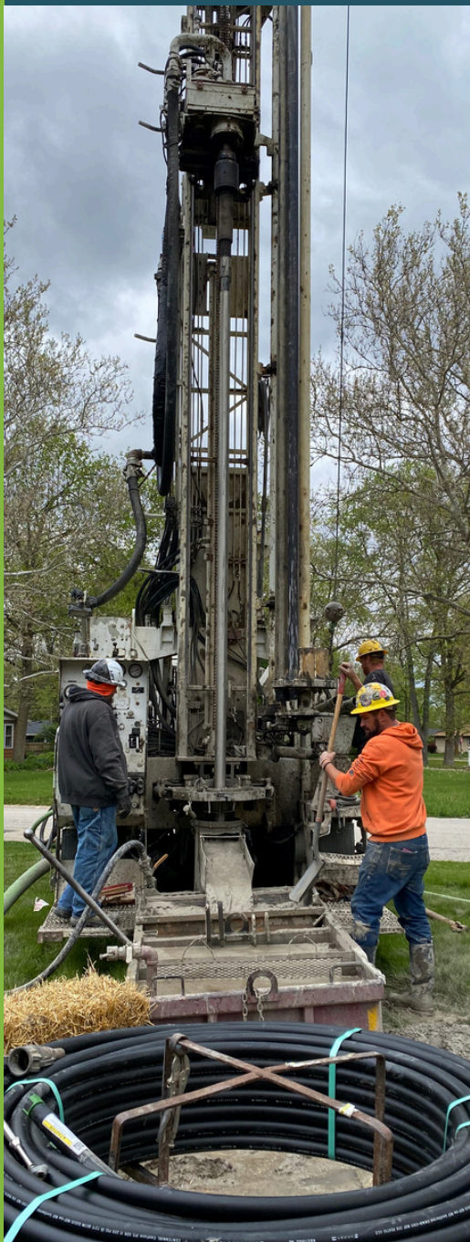
Photo: Geothermal Well Drilling
