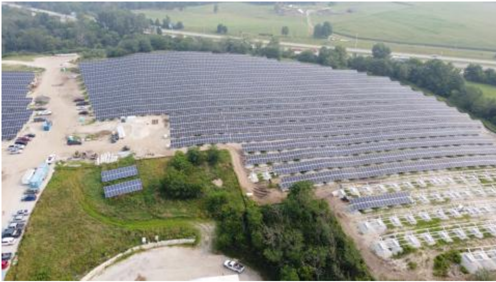
City of Urbana Community Solar Array
