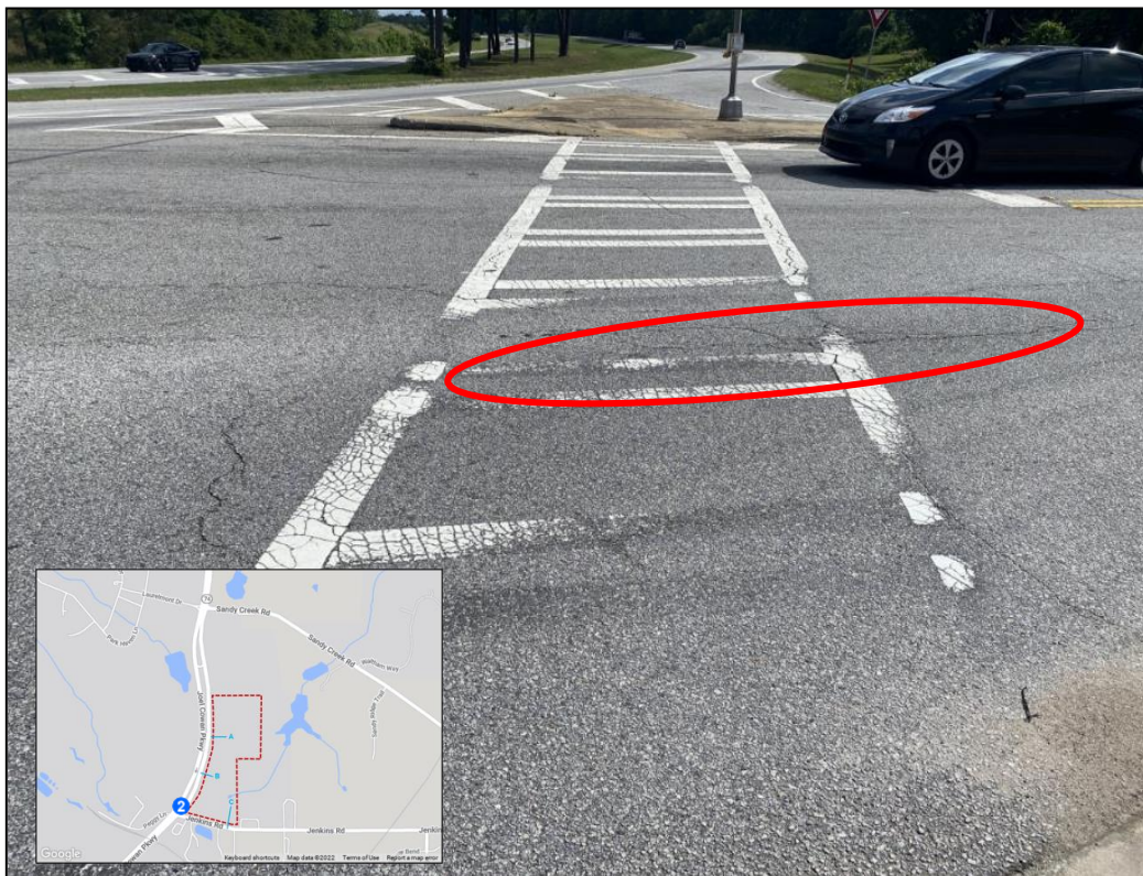
Figure 5: Eastbound/Westbound Jenkins Road Minor Pavement Cracking
