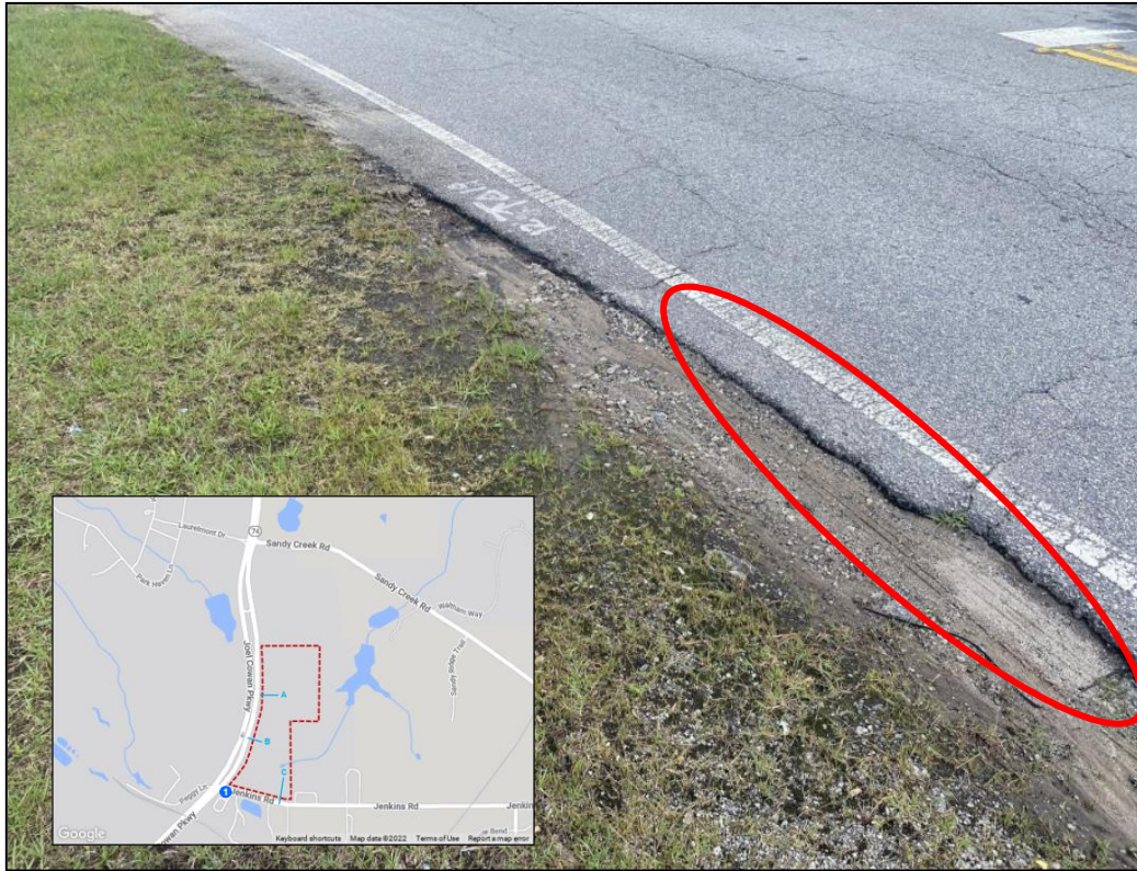
Figure 4: Eastbound Jenkins Road Shoulder/Pavement Cracking
