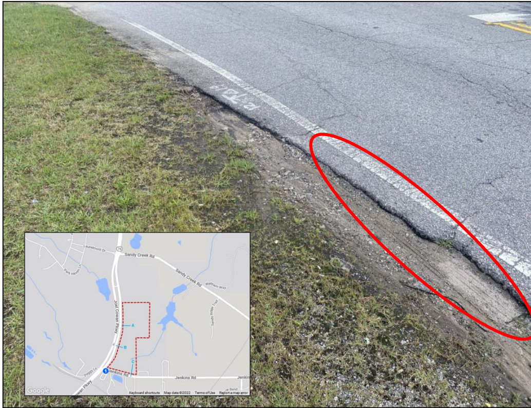
Figure 4: Eastbound Jenkins Road Shoulder/Pavement Cracking
