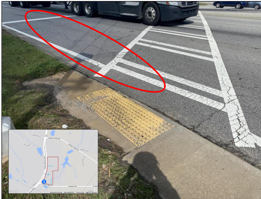
Figure 6: Northbound Joel Cowan Parkway (SR 74) Minor Pavement Cracking
