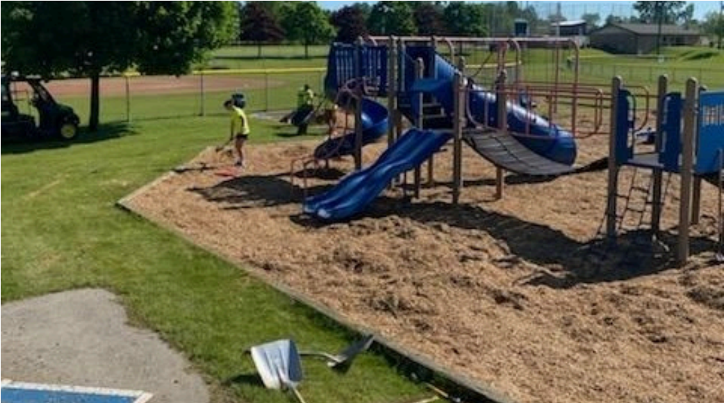
New mulch being installed at the playground.
