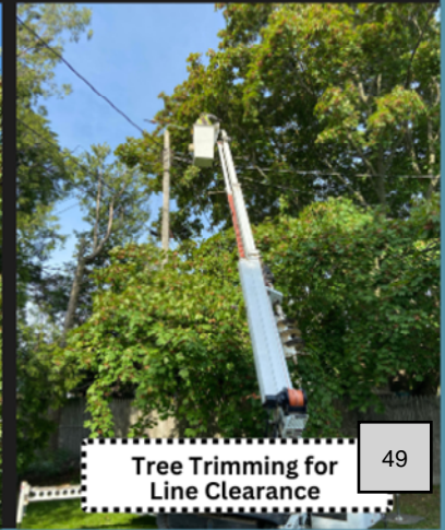
Tree Trimming for Line Clearance
