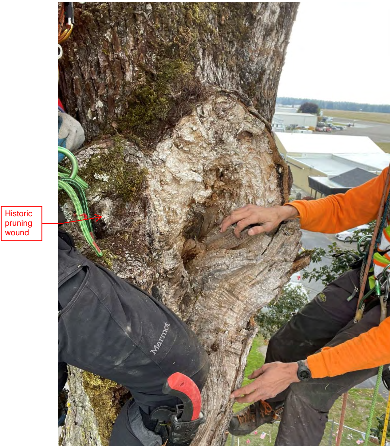
Figure 13 Additional view of 2023 failure and historic pruning wound.
