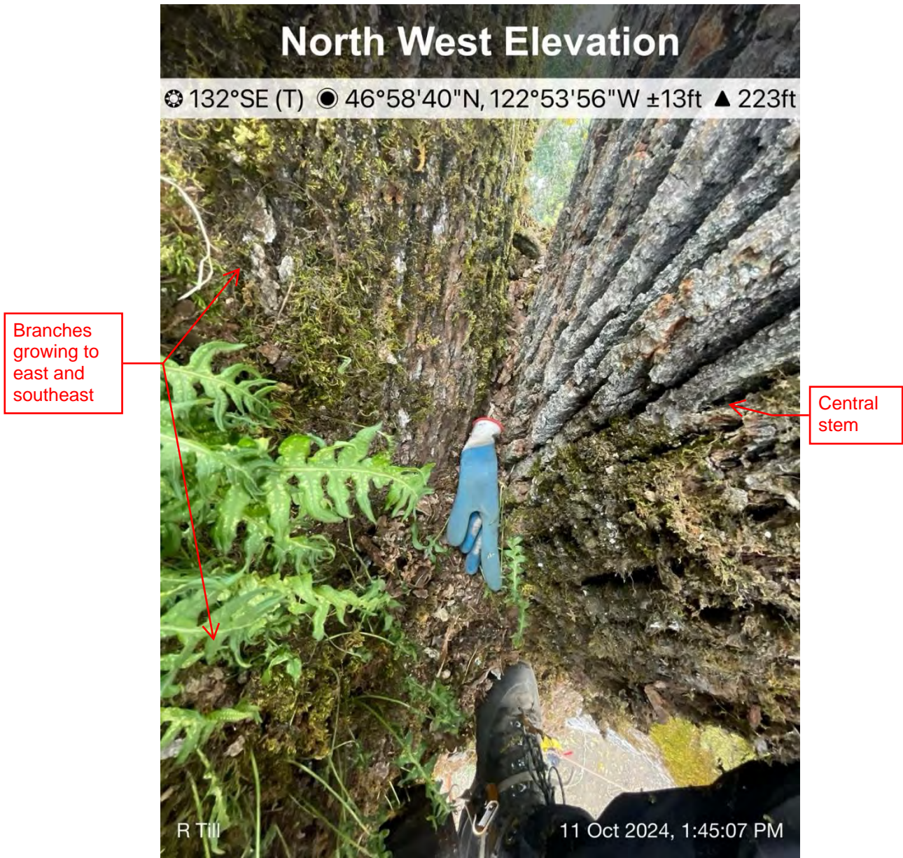
Figure 6 View directly down into second codominant union. Two stems over the road are on the left and central stem to the right. Union has included bark. Probing did encounter solid resistance beneath debris.
