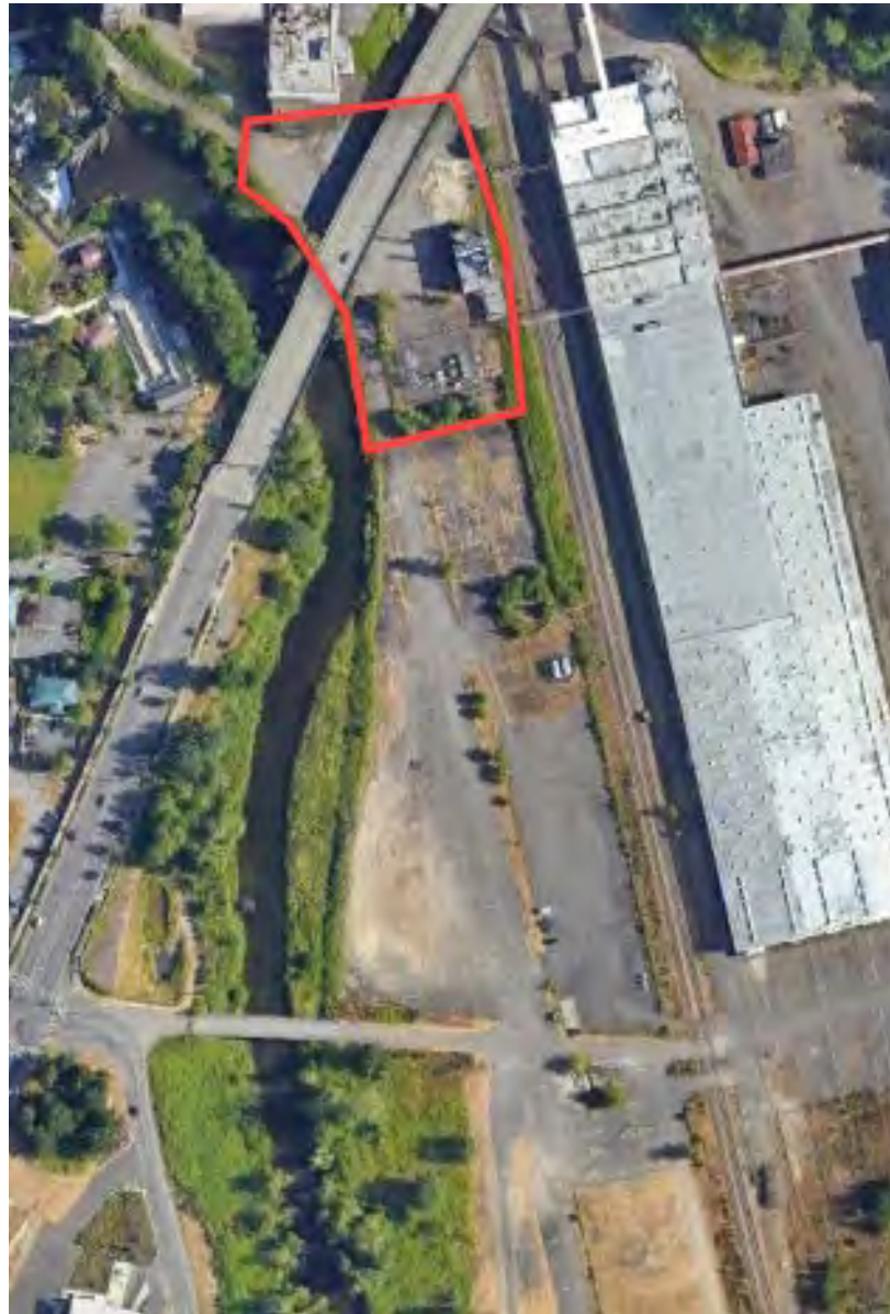
Figure 33 – Power Substation and Ground under Capitol Blvd Overpass to be Lowered
