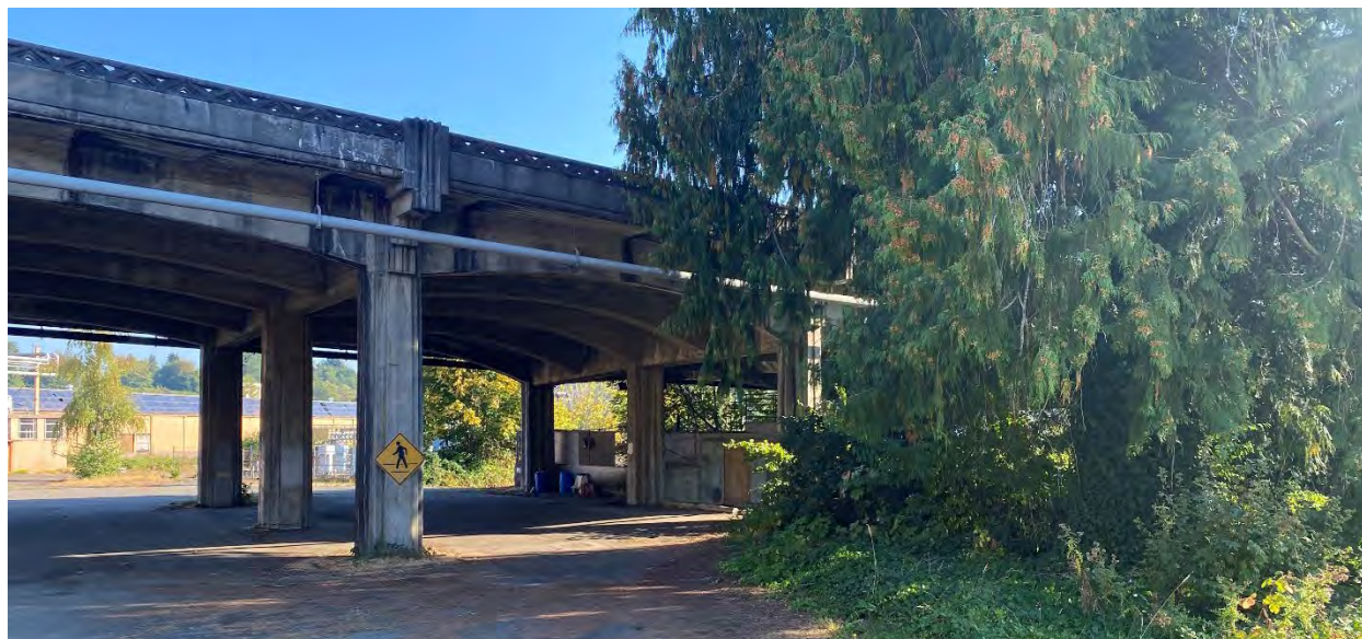
Figure 10 – Image of Capitol Blvd Right Overbank
