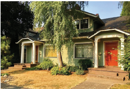
Duplex (side-by-side) in Everett, WA
