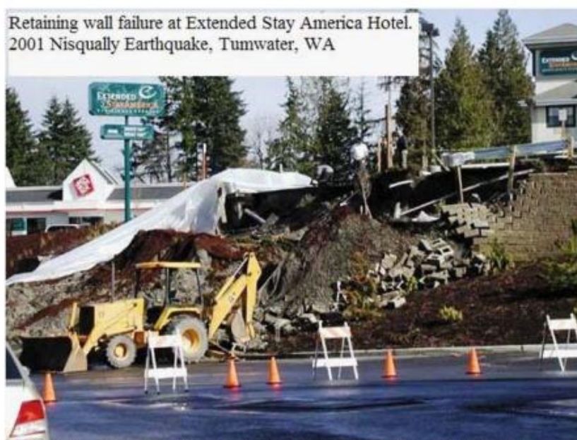
Figure 2: The Extended Stay America facility near the Highway 101/Crosby Boulevard interchange had a large retaining wall give way, which broke a water line (Former Tumwater Fire Chief John Carpenter-phone conversation 6-3/9/10-2009)
