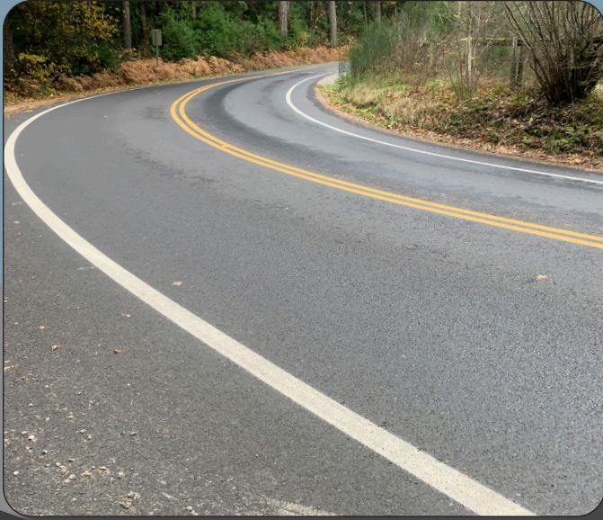
83rd Avenue at Armstrong Road
