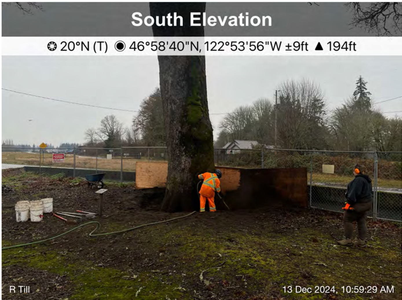
Figure 1 Root crown excavation employed an “air spade” that uses compressed air to remove fine soil. The excavation involved alternating between air spade removal of soil with hand removal of river cobble that was backfilled over the root flare after a prior root crown excavation. The project archaeologist oversaw all work.
