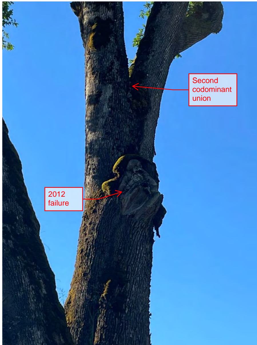
Figure 3 2012 failure and the second codominant union related to the following series of photos.
