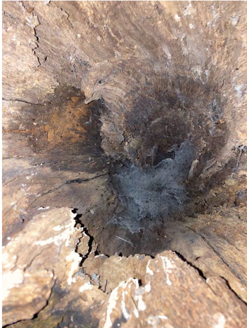
Figure 24 View vertically up the cavity.
