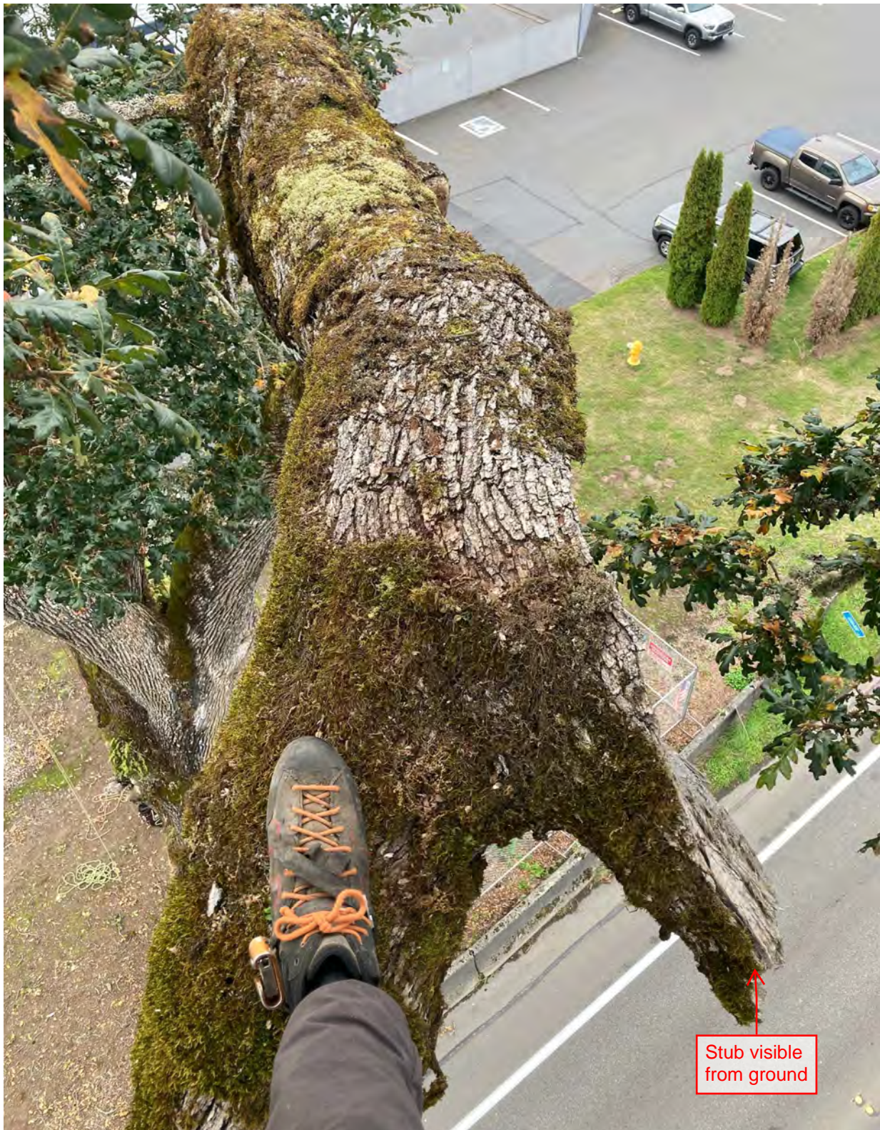
Figure 26 View from above failure showing extent of sound wood supporting remaining stem.
