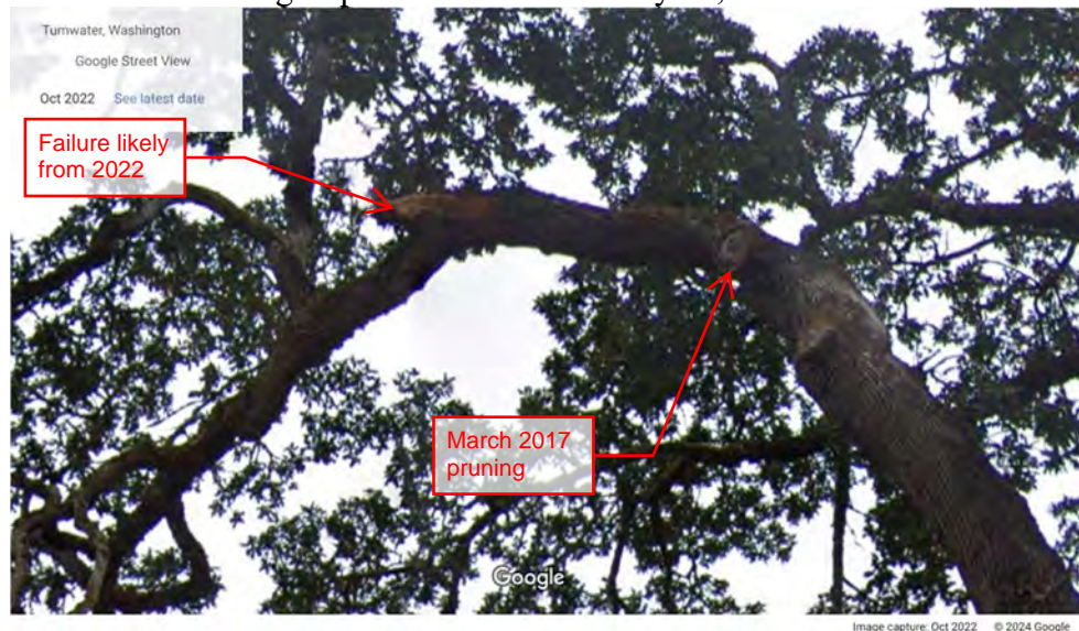
Figure 4 October 2022 view of branch over Old Highway 99.
