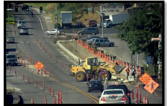
This 2014 Capitol Way project added bike lanes and improved the sidewalks in this part of the Brewery District in addition to improving stormwater runoff facilities.
