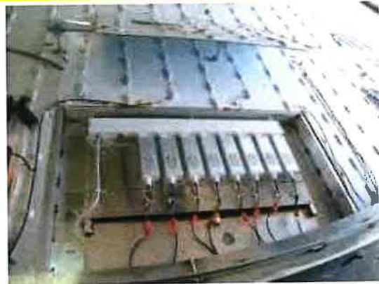
Service access centered at bottom for electric hook-up and maintenance at bottom/back of sign.
