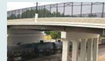
Tualatin-Sherwood Road bridge over Boones Ferry Rd
