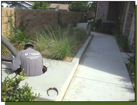
Vacuuming out of media filters.
