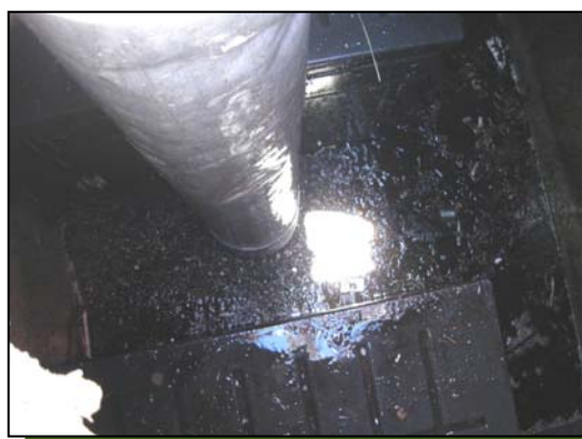
Removal of trash, sediment and debris.
