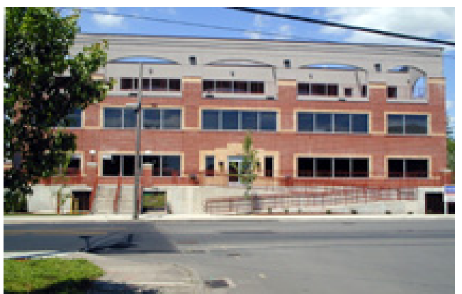
Aspen Place – Boones Ferry Road
