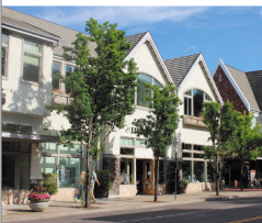
DO Establish a higher percentage of frontage along key corridors to promote a highly walkable pedestrian environment.
