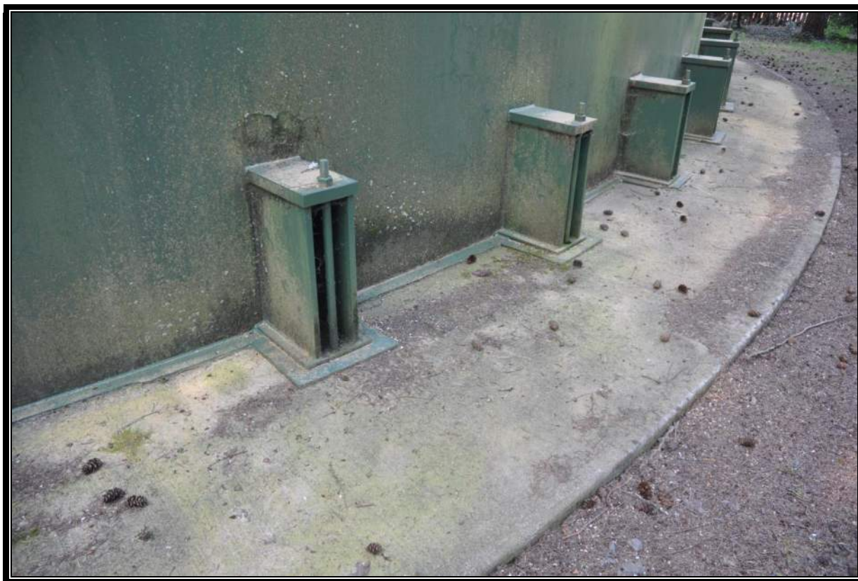
2.2 MG A1 Reservoir – Foundation and Anchorage Retrofit
