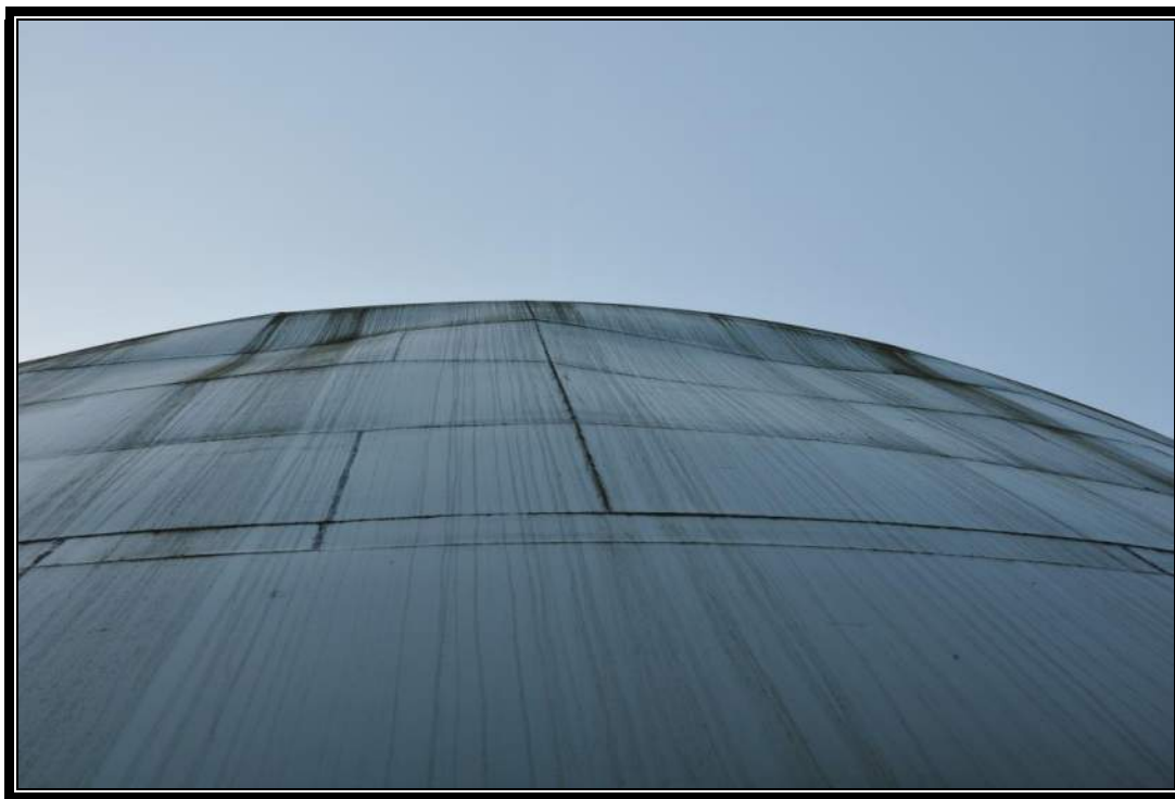
2.2 MG B1 Reservoir – Wall Shell Plate Buckling
