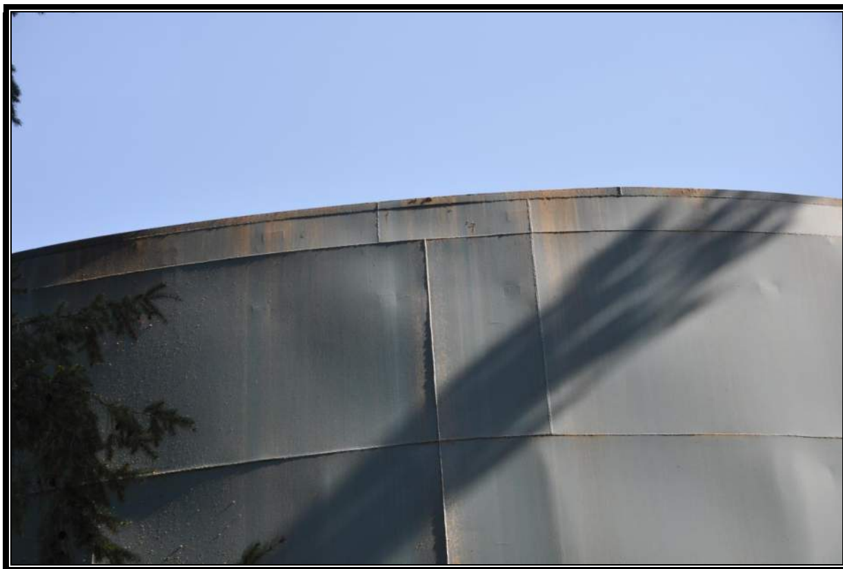
2.2 MG A1 Reservoir – Buckled Wall Shell Plates
