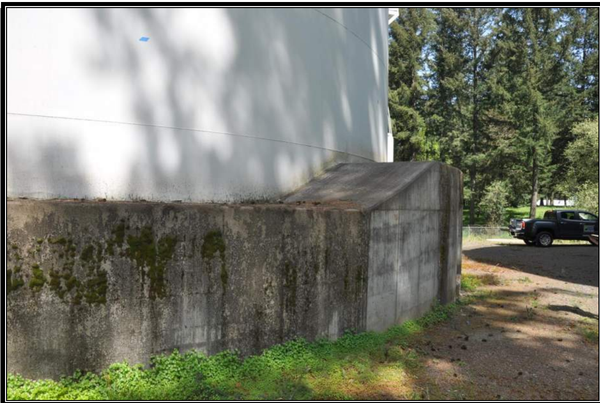
0.8 MG C1 Reservoir – Ballast Ring
