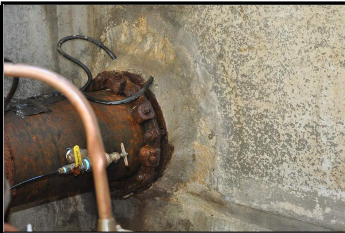
Boones Ferry Control Station – Rigid Pipe Penetration Through Vault Wall
