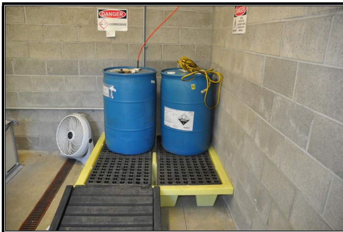
ASR Pump Station – Unbraced Chemical Barrels
