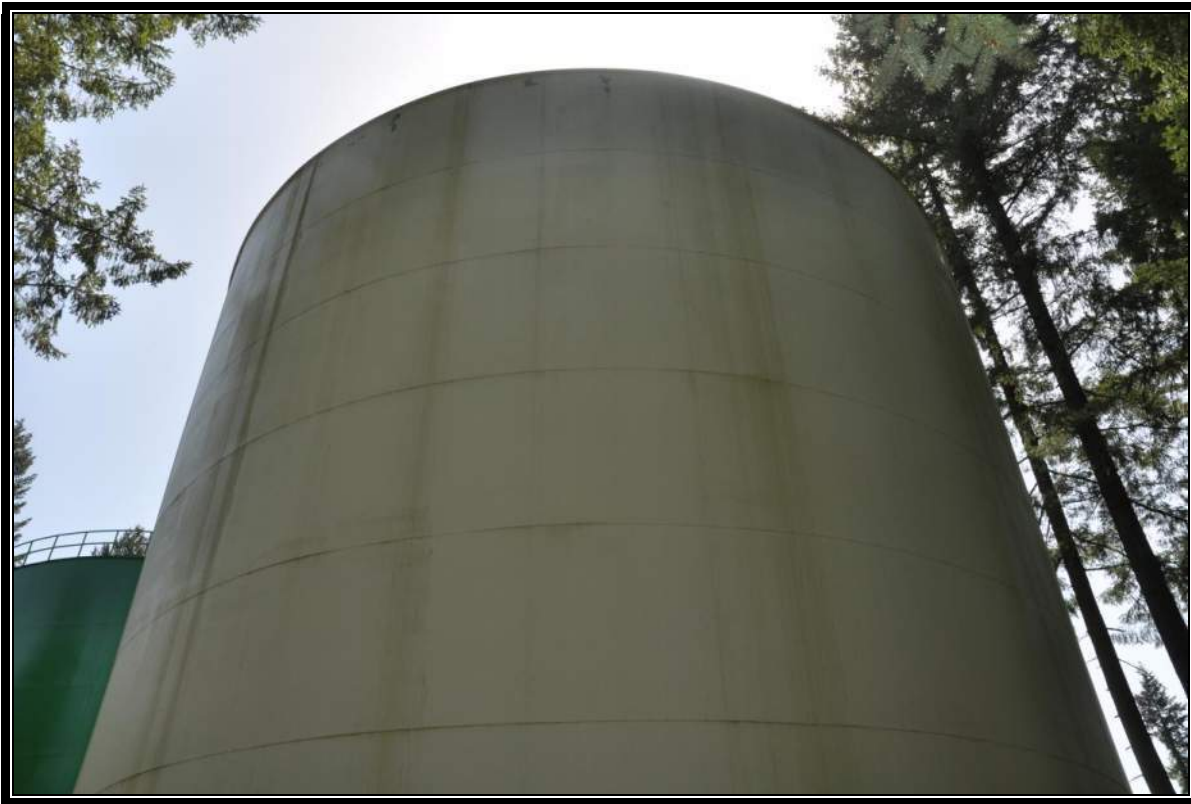
0.8 MG C1 Reservoir – Wall Shell Plates
