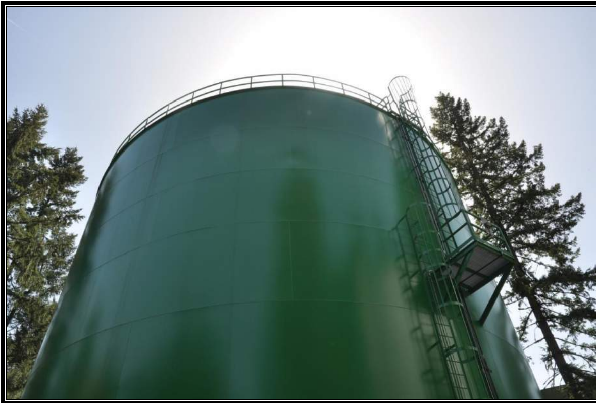
1.0 MG C2 Reservoir – Wall Shell Plates
