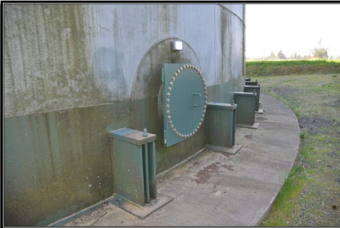
2.2 MG B2 Reservoir – Anchorage Retrofit
