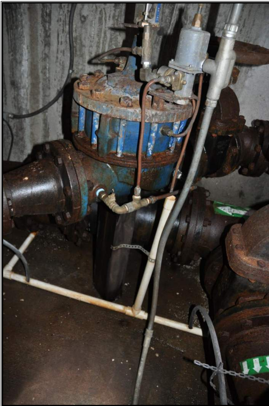
Martinazzi Pump Station – Outdated Pipe Bracing
