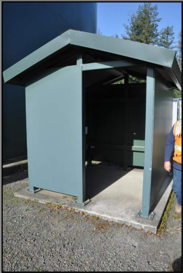
5.0 MG A2 Reservoir - Shelter
