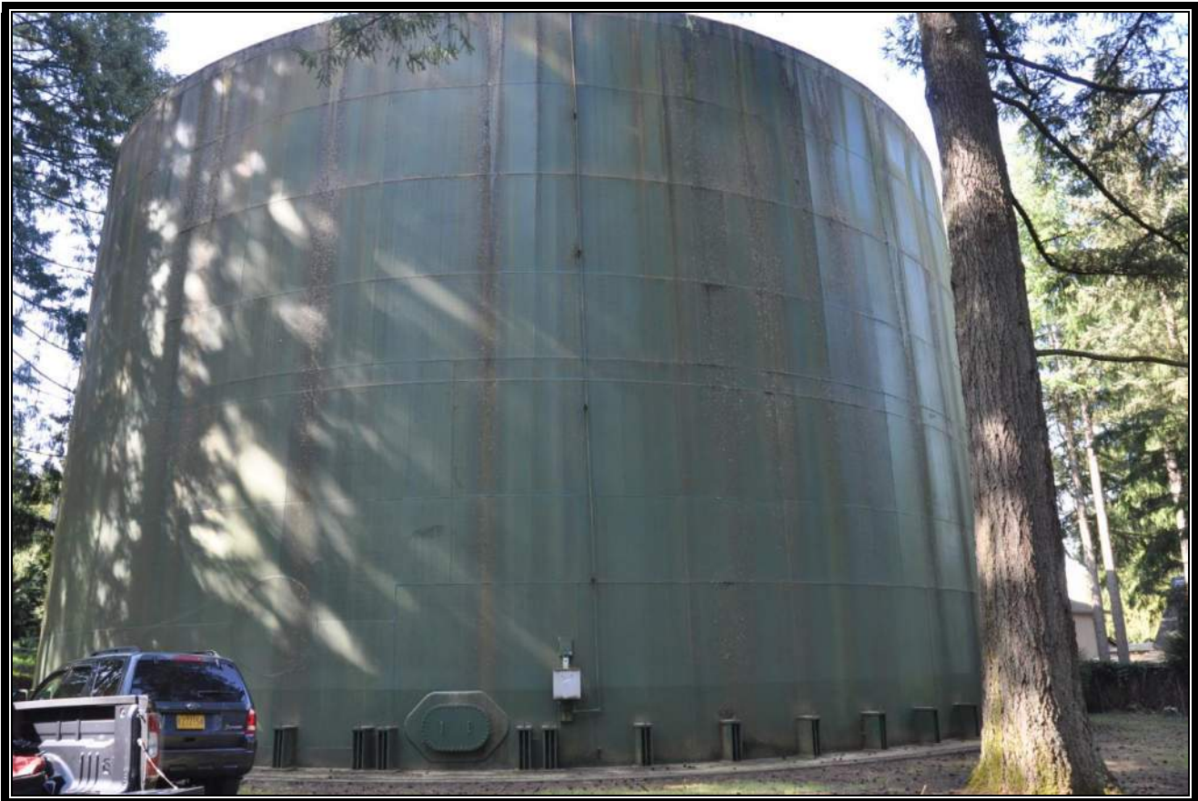
2.2 MG A1 Reservoir
