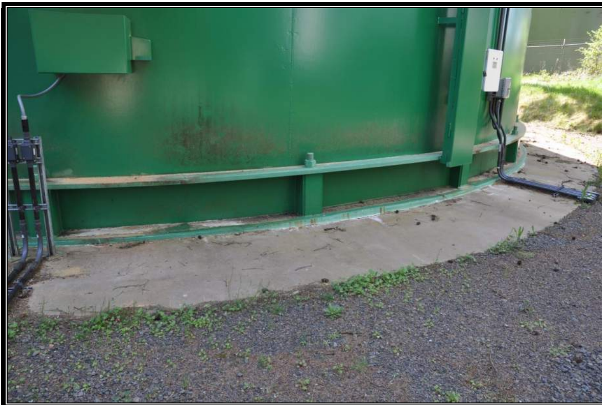
1.0 MG C2 Reservoir – Anchors and Foundation
