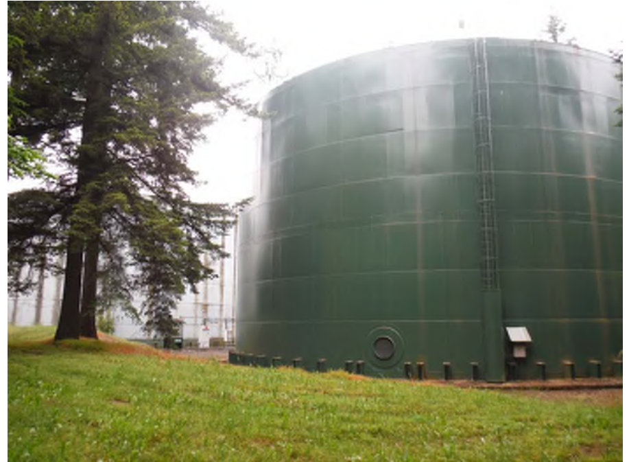
Photo 6: Norwood reservoirs and pump station, looking west (May 30, 2018).
