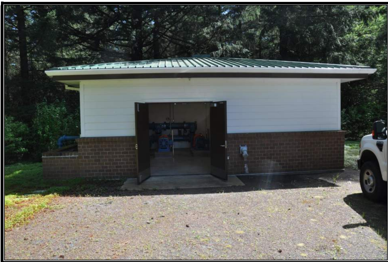
C Level Norwood Pump Station
