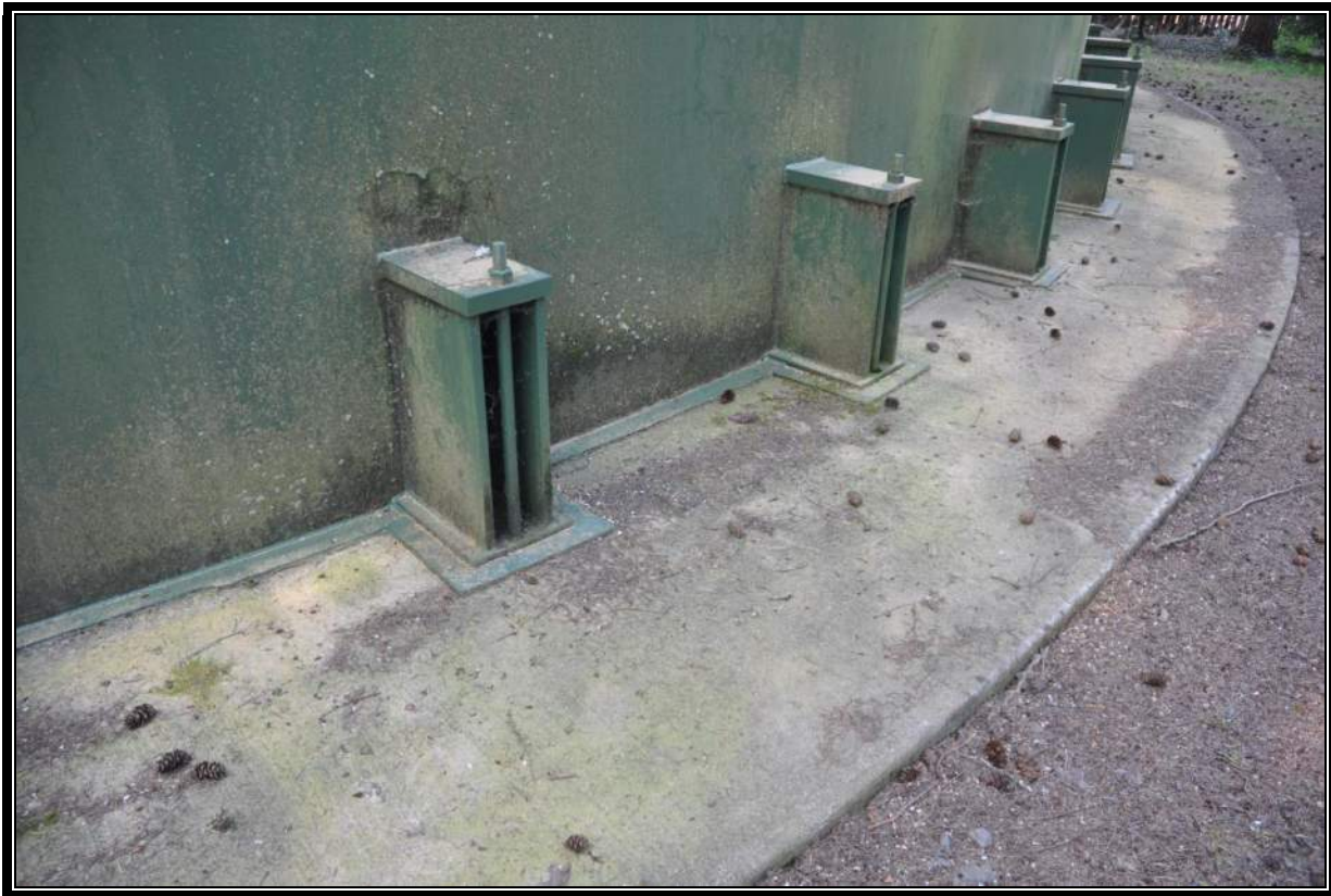
2.2 MG A1 Reservoir – Foundation and Anchorage Retrofit
