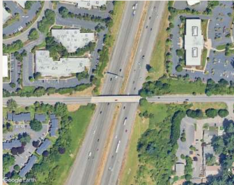
Sagert Street Bridge Lights
