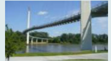
65 th Avenue Bridge
