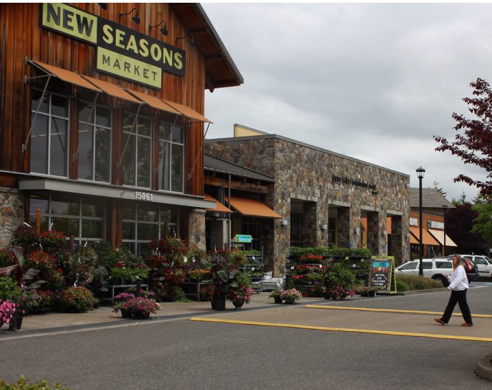
DO Require more than just paint striping to demarcate pedestrian walkways.
