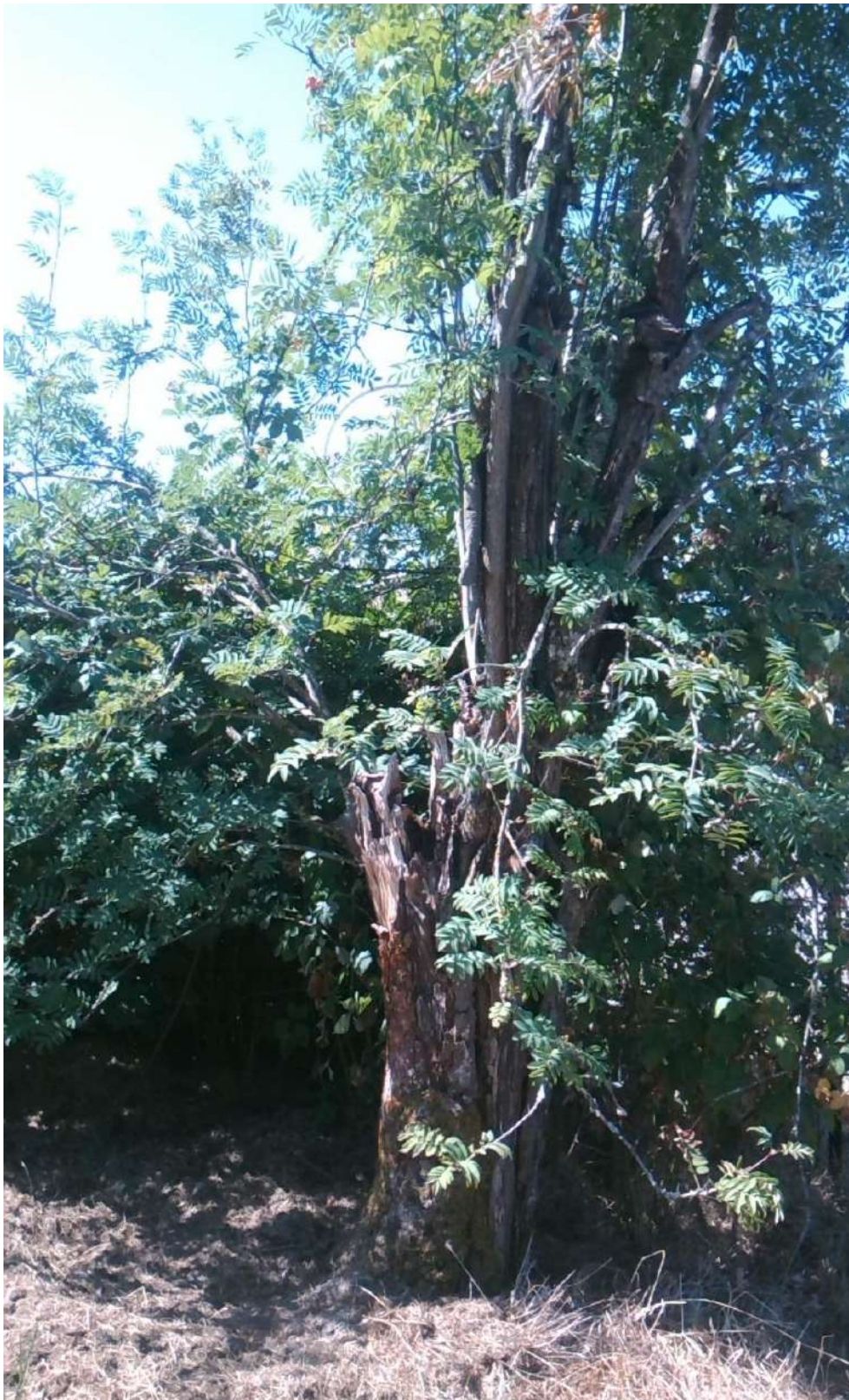
Photo 2. Tree #34 is a mountain ash that is hazardous to preserve due to previous failure, crack, and weakly attached epicormic shoots. It meets the conditions of TDC 33.110 (5)(a)(ii)(B); substantial portions of the tree are in danger of falling.
