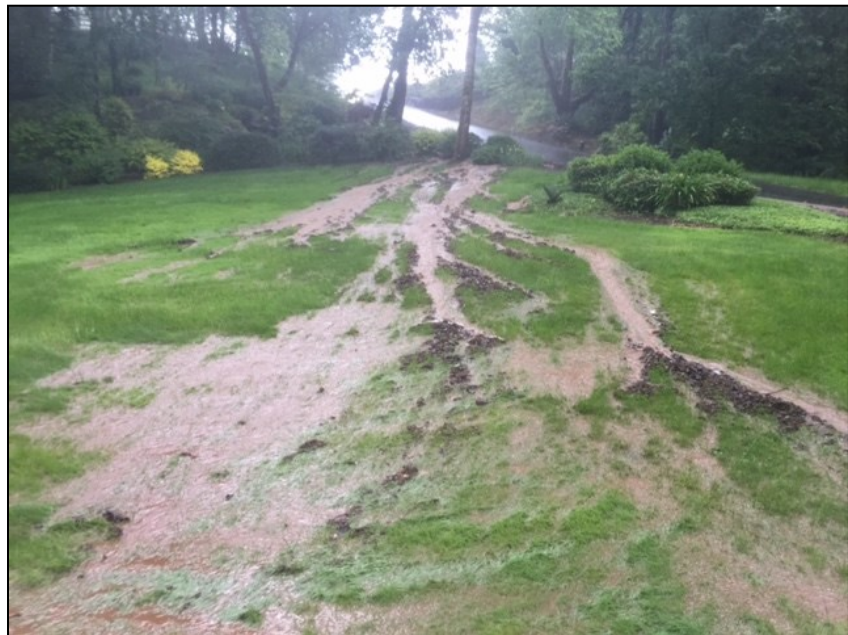
Photo A2d. Flooding storm water ultimately found its way onto the porch and steps of the house and into the lower driveway area (5-18-15).
