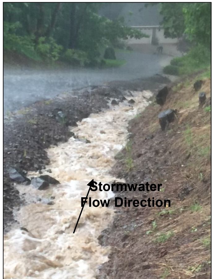
Photo A2b. Channel conveying Boones Ferry Road drainage across the Lucini property (5-18-15).
