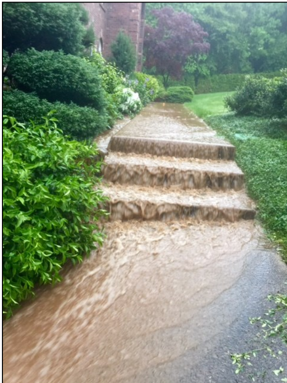
Photo A2f. The front walkway steps drain into the lower driveway and garage area.
